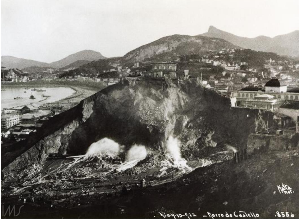
Figure 12: The Morro do Castelo, or Castelo Hill, being removed in 1922. The world's fair happened where the hill used to exist. Photo by Augusto Malta, Brasileira Fotografia.
