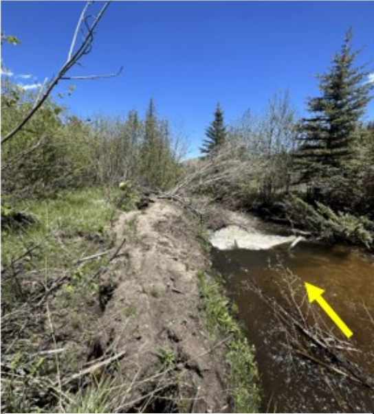
Large block failure of left bank at fourth bead on Little Beaver Creek. Felled bank trees have created local knickpoints; tree conditions suggest this failure is recent.
