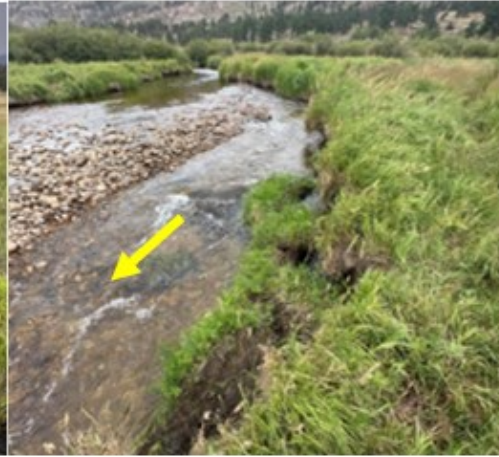
Bank collapses on river left on the Big Thompson River at Moraine Park, RMNP.
