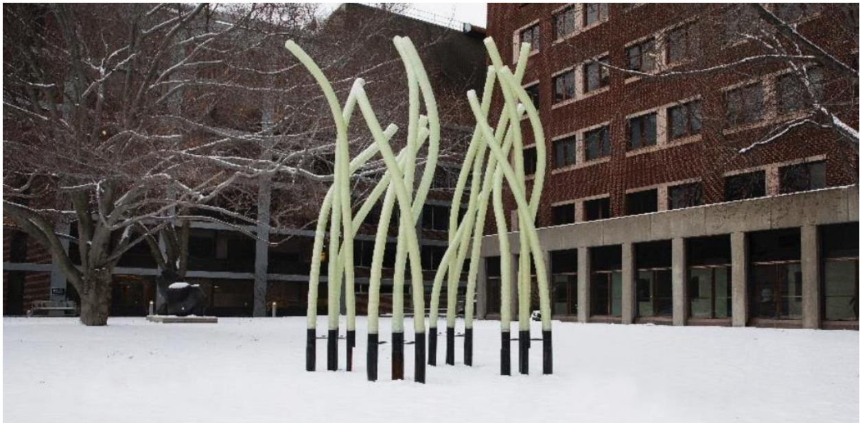
Figure 1-6: Large fiberglass reinforced structure created by Fiberbots [30].
