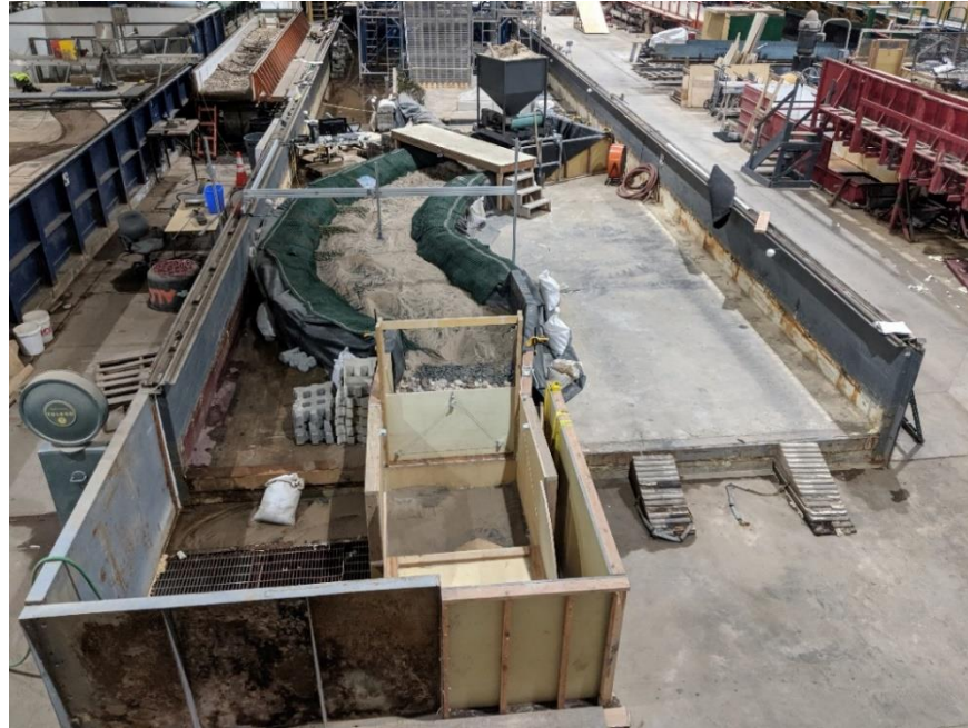
Figure 23: A view of the completed curved flume. The view also shows a configuration of BW's placed in the flume.
