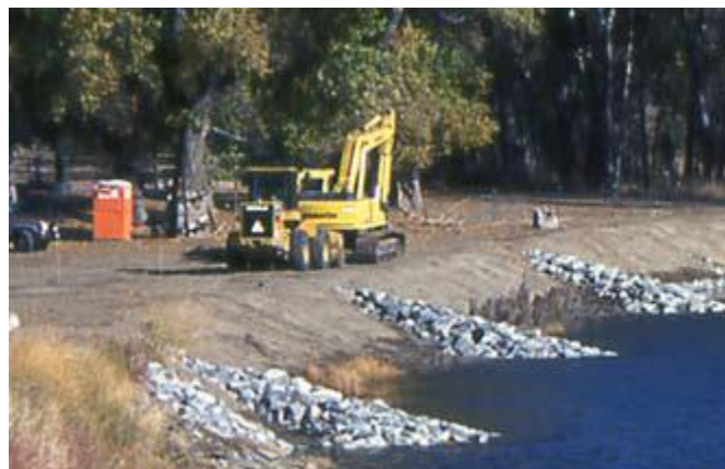
Figure 3: Installation of rock vanes (NRCS 2007)
