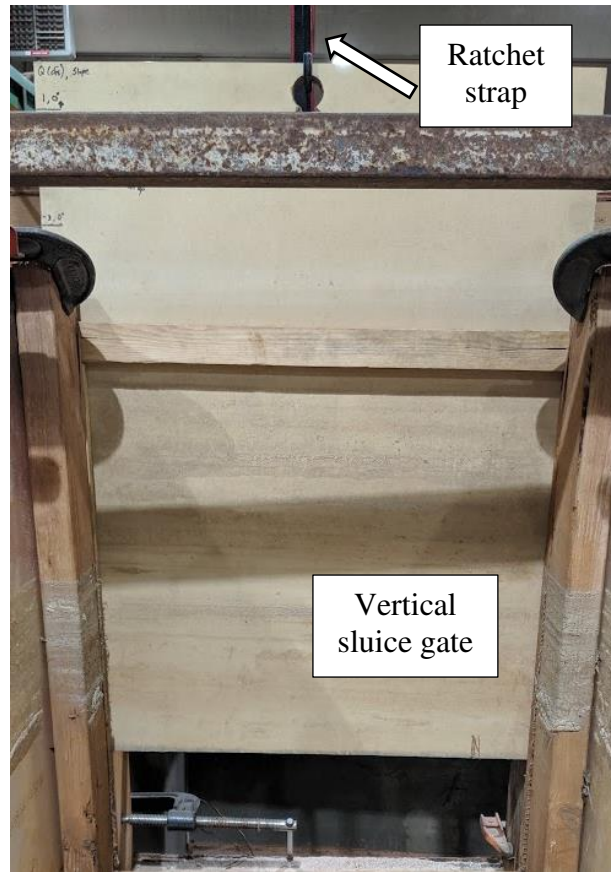
Figure 9: The vertical sluice gate used at the downstream end of the straight flume. The strap-controlled flow along the flume
