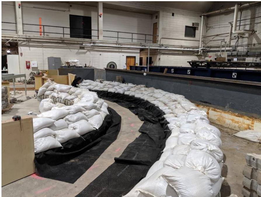
Figure 20: Completed curved flume channel walls without the rubber pond-liner and the Pyramat® cover. This figure shows how the flume's curved channel was built
