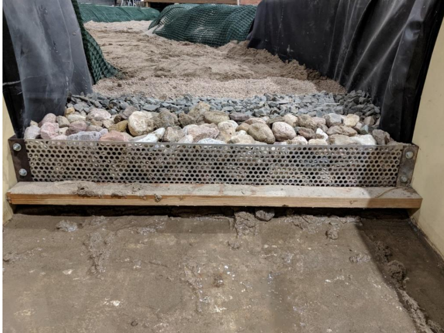
Figure 26: Upstream view of riprap and drainage at the downstream end of the flume's curved channel
