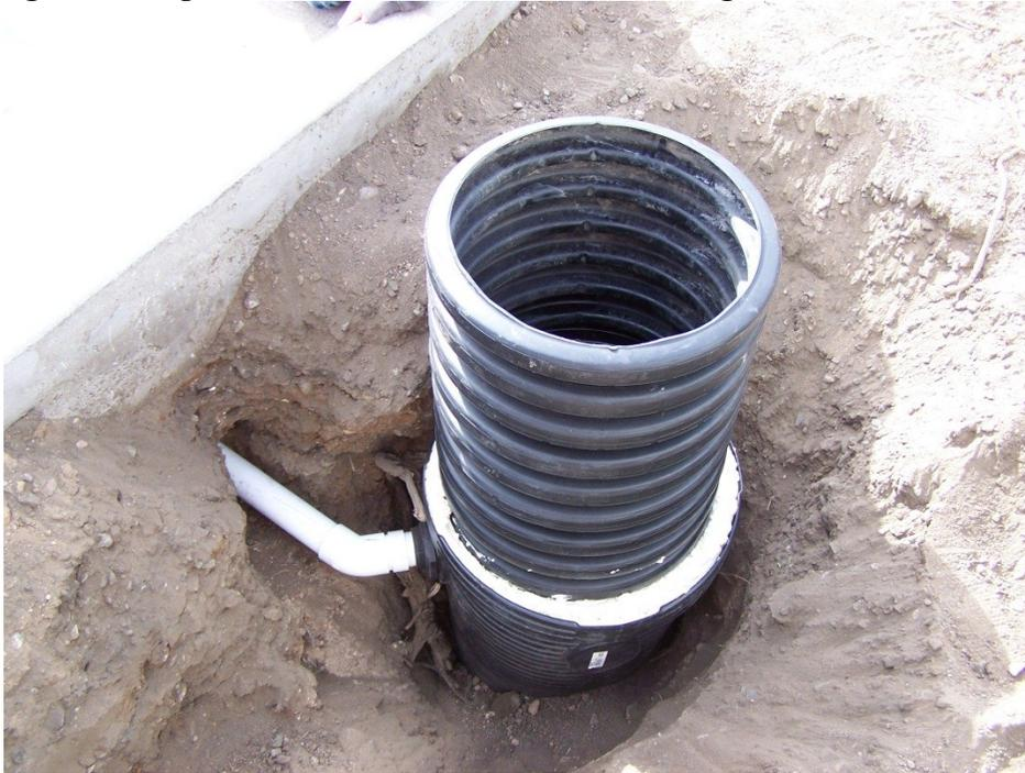
**Figure 10: Installation of water quality sump with under-drain connection at CTL PL**
