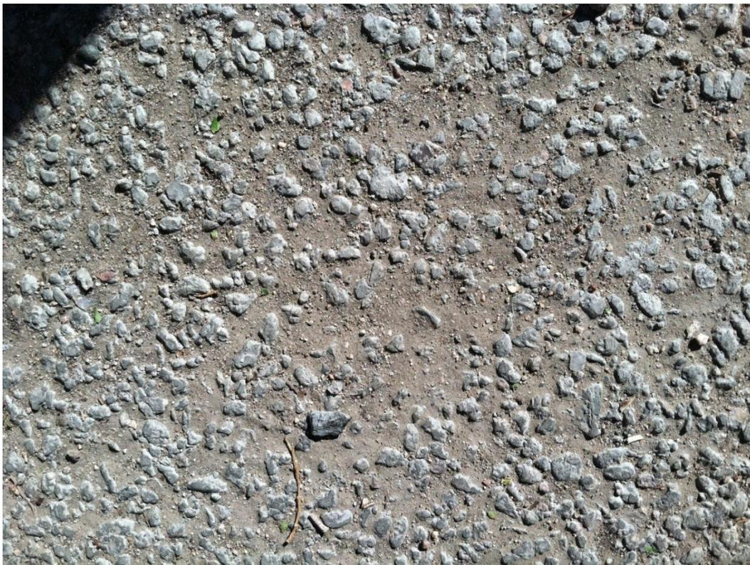
**Figure 19: Clogged section of the CTL PC Parking Lot**
