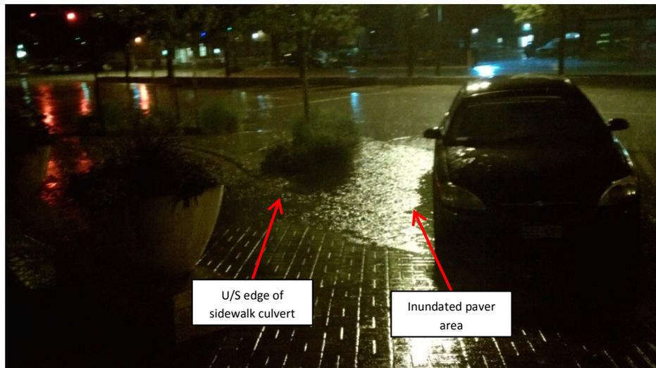
**Figure 22: Severely inundated pavers during storm due to clogged culvert**
