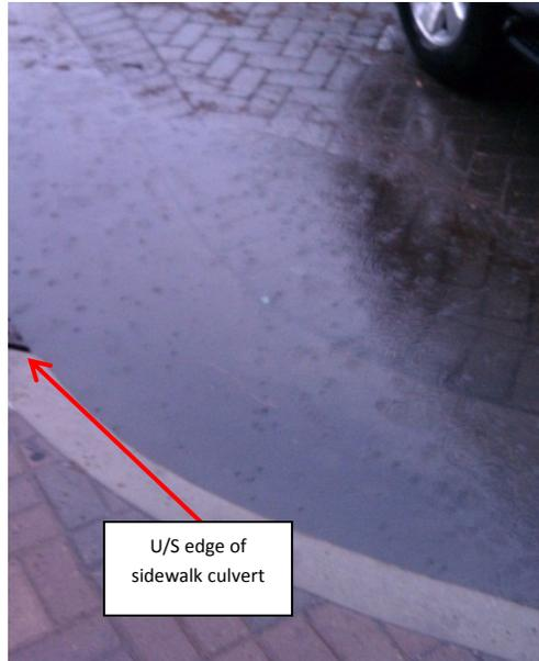
**Figure 21: Flooded pavers during storm due to clogged culvert**
