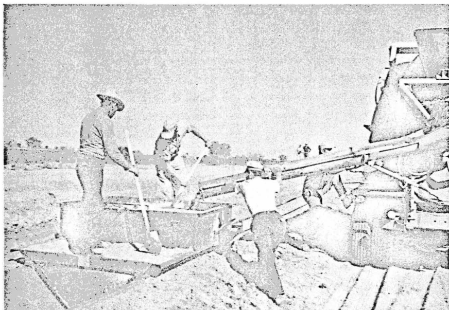
Figure 14—Casting two-inch concrete lining with a slip form. Form is pulled on long hitch by tractor.
