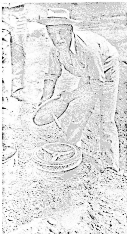
Figure 39—An alfalfa valve being set on a concrete riser pipe.
