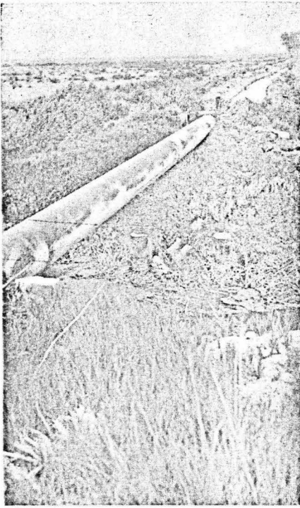
Figure 31—Unsupported plain steel pipe flume.
