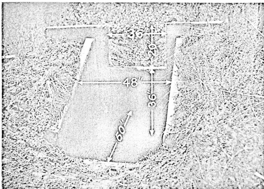
Figure 21—A well proportioned two-foot concrete drop.
