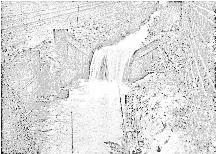
Figure 22—V-notch timber drop. A horizontal crest would have reduced the depth of overpour and the downstream wall should have had a wider opening. Timber structures are subject to fire damage.
