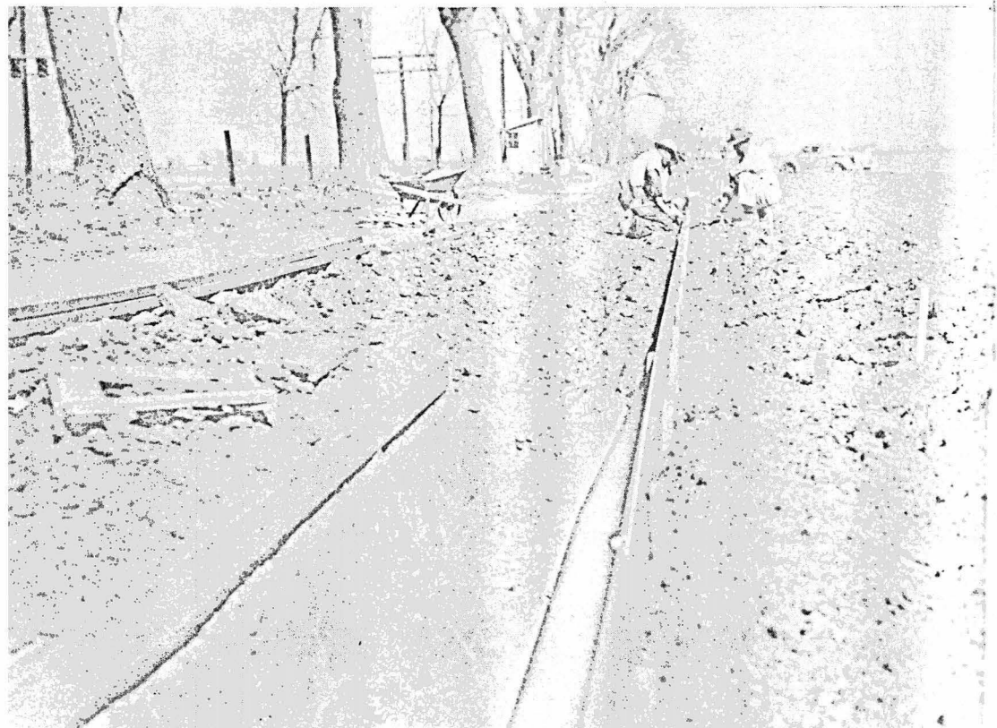
Figure 7—Setting guide rails for concrete ditch lining. Rails serve as a guide on which an excavation template (arrow) rides as an outside form for the top of the lining and as a support for the inside forms.
