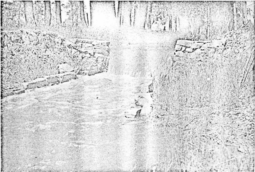
Figure 23—Use of masonry for a drop.
