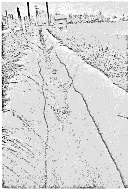
Figure 11—A 3-inch concrete plaster lining 15 years old.
