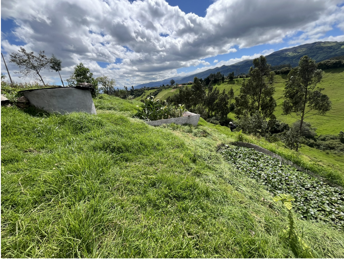
Figure 11: Pintag Amaru's biofiltration system, cleaning their gray and black water before sending downslope.
