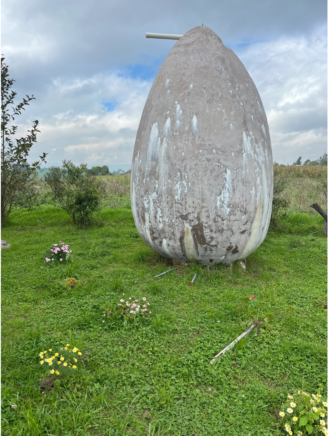
Figure 10: Pintag Amaru's rainwater collection system
