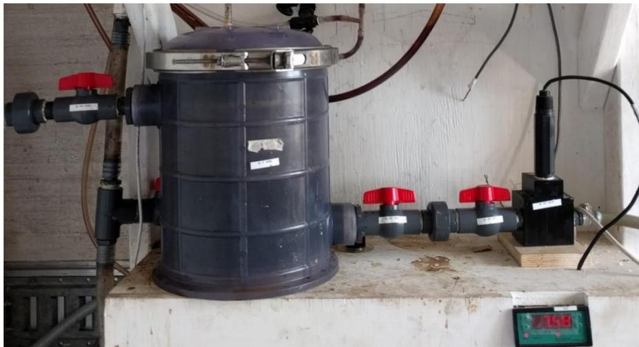
Figure 21. FFR leachate pre-filter and inline pH transmitter
