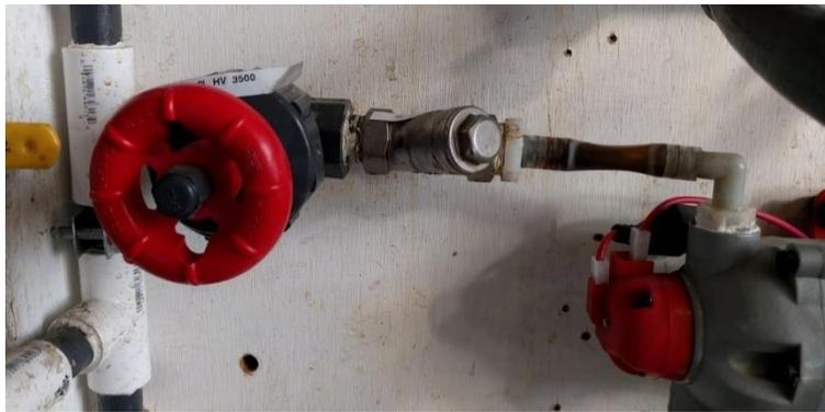
Figure 15. Detail of LBR pump manifold valve and inline filter.
