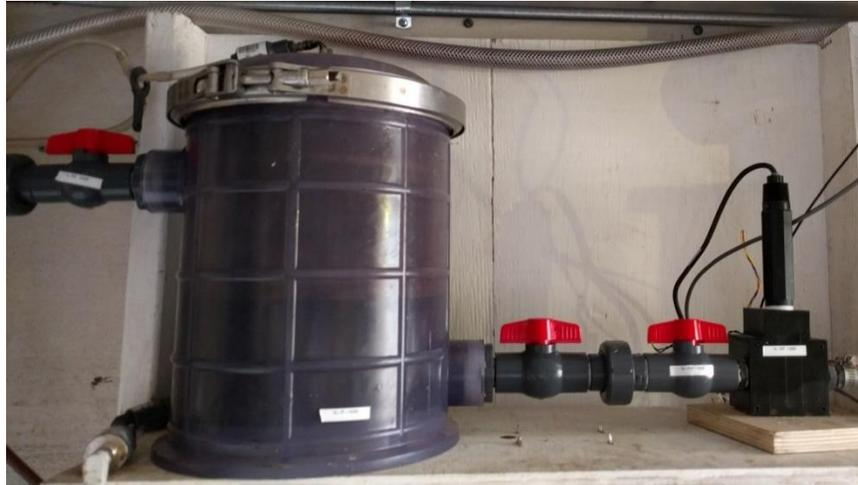
Figure 13. LBR pre-filter- PurFlo 10 micron pleated filter.
