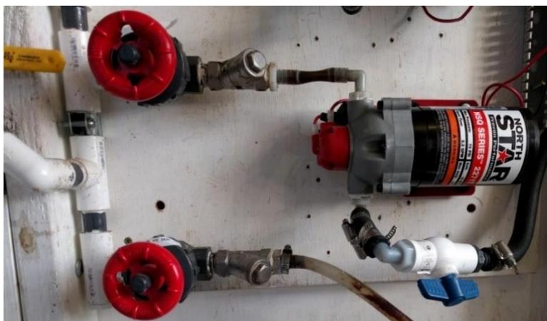
Figure 22. FFR leachate delivery pump (top valve) and leachate sample port (bottom valve)
