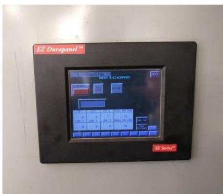
Figure 11. Human machine interface- EZ automation EZ Dura-panel 6.”
