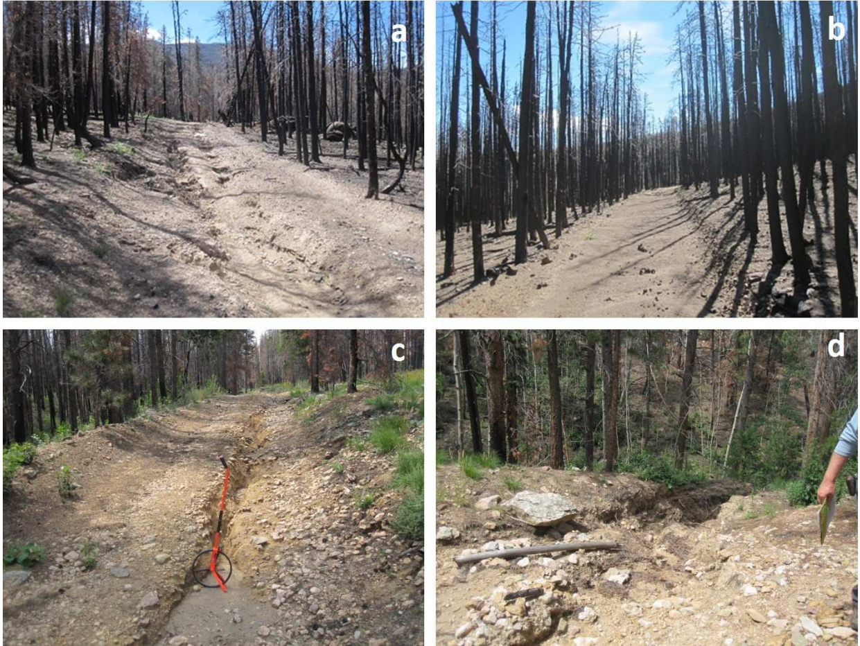
Figure 1.4. Representative road segments along Old Flowers Road. a) Road segment with 10% slope and road surface rilling below an area that burned at high severity. b) Road segment with only 2% slope below an area burned at high severity with no rills due to deposited sediment. c) Road segment below an area that burned at moderate severity showing how the one rill in the wheel track closest to the upper side of the road captures all of the runoff from the burned hillslope above the road. d) Single, deeply incised gully leaving a 51-m long road segment that was in an area that burned at high severity. This gully extended at least 10 m to the ephemeral stream at the base of the slope, and the large size of this drainage feature can be attributed primarily to the combination of runoff from the burned hillslope and the 15% slope of the road segment.
