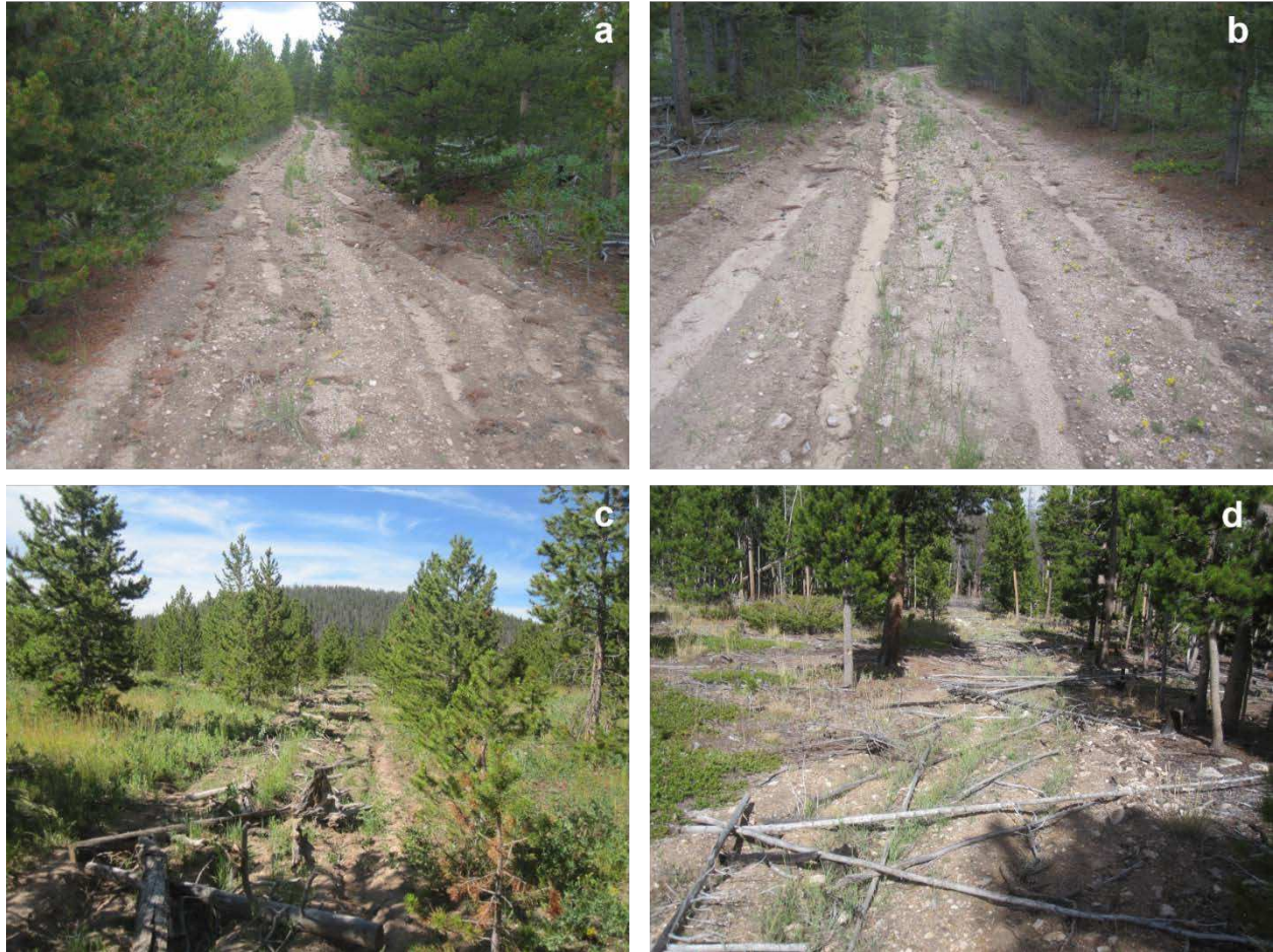
Figure 3.8. Typical road segments one year after decommissioning. a) Segment with 4% slope that was only ripped. The road surface shows evidence of erosion, but all of the eroded sediment was trapped in the furrows created by the ripping. b) Segment with 9% slope that was only ripped, showing much more eroded, transported, and deposited sediment. c) and d) Road segments that were ripped and mulched showing much less erosion due to the mulch plus greater vegetative regrowth and slash cover compared to the segments that were only ripped.
