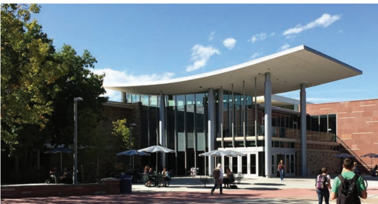
Lory Student Center Renovated May 2013- September 2014
