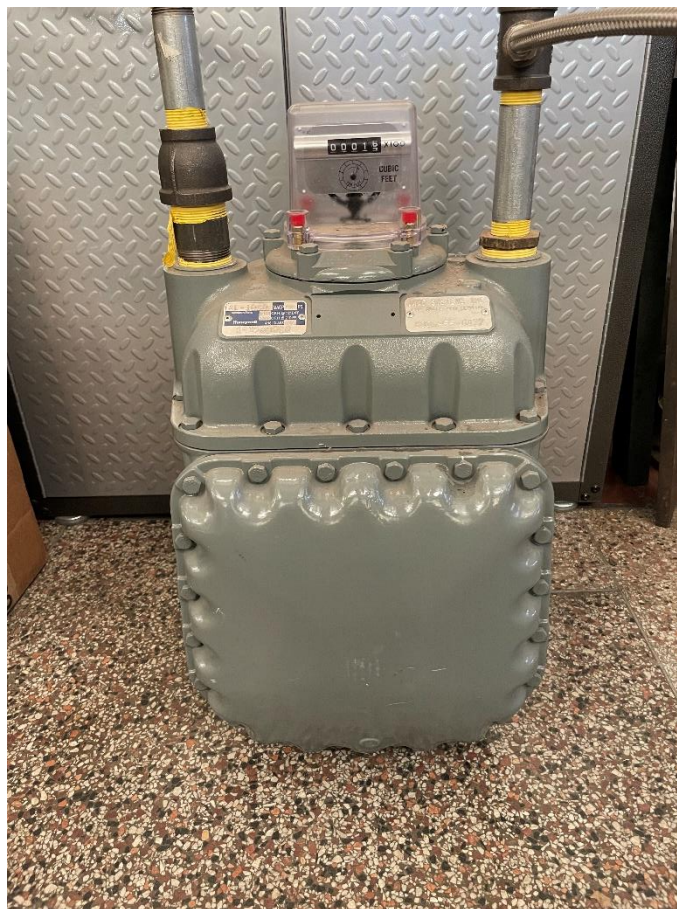
Figure 40: 1ft 3 -Positive Displacement Gas Flow Meter
