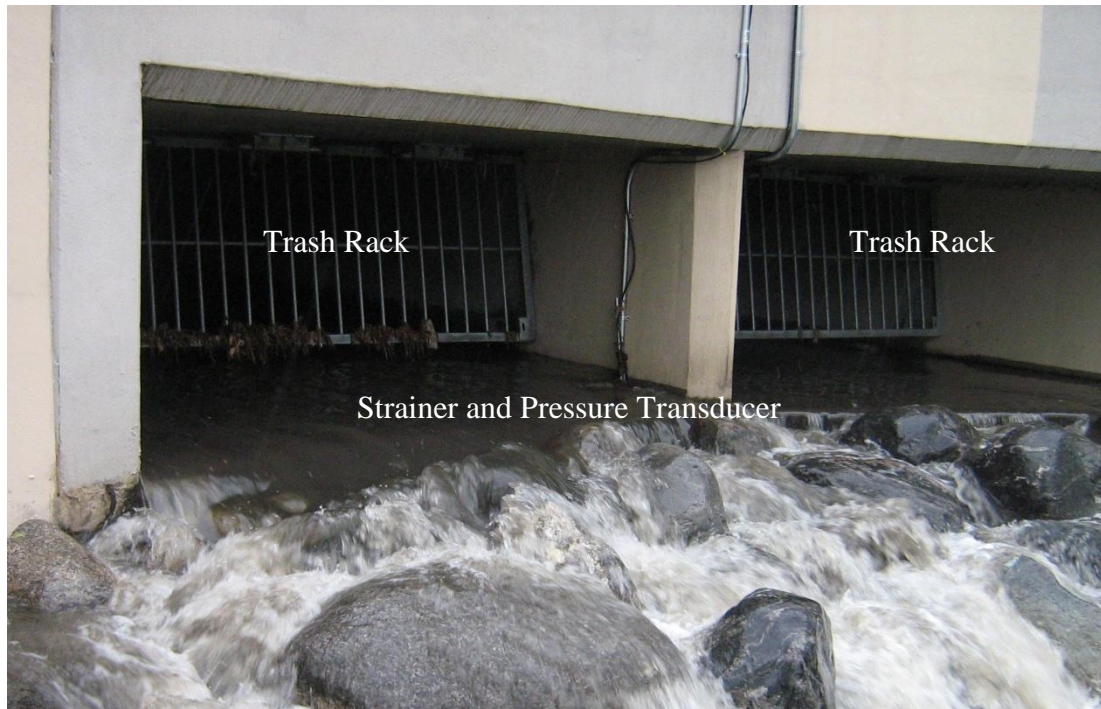
Figure A-8. Howes St. Inlet Configuration
