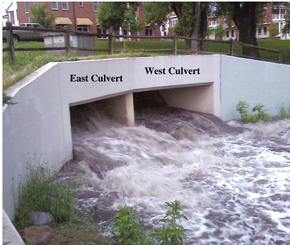
Figure A-7. Uneven Discharge for the Howes St. BMP Inlet
