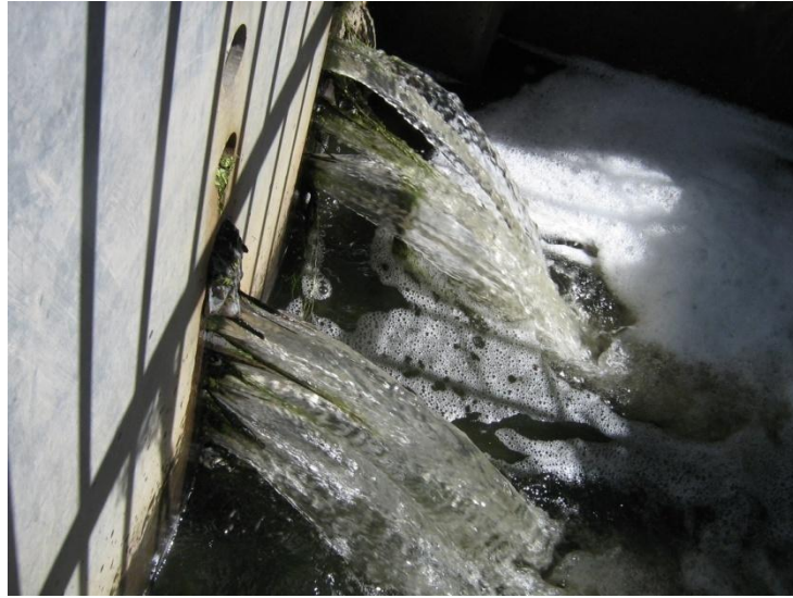
Figure A-3. Water Flowing through Orifice Plate at Pond 2
