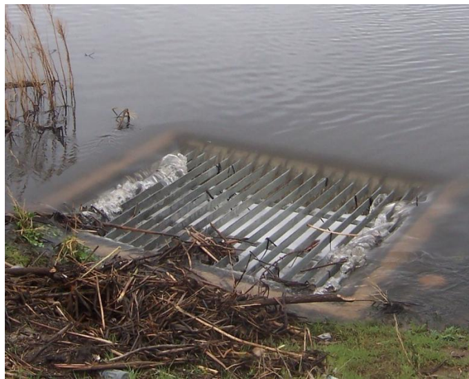
Figure A-4. Water Flowing through the Trash Grate at the Pond 1 Outlet Structure
