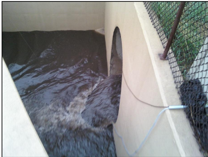
Figure A-1. Overhead View of Runoff Entering the Udall WP through the Inlet Pipe
