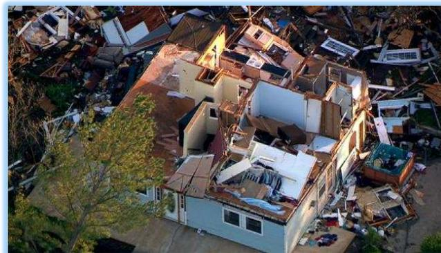
**FIGURE 2. 9 – Typical roof-wall connection failure (newsons6.com)**
