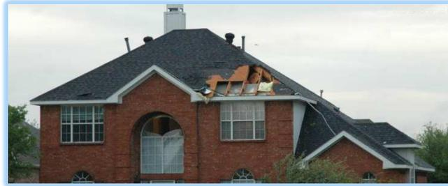
**FIGURE 2. 8 – Typical roof panel failure (RoofingAnnex.com)**
