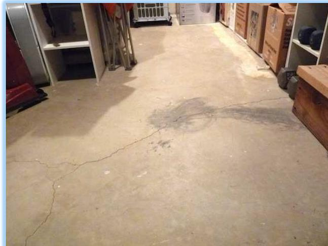
**FIGURE 2. 13 – Typical foundation slab cracking due to expansive soils (nachi.org)**
