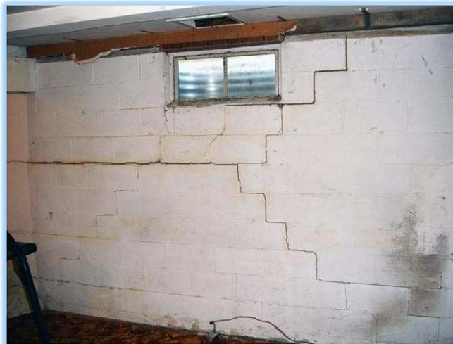
**FIGURE 2. 12 – Typical masonry basement wall cracking due to expansive soils
