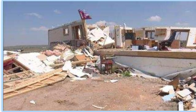
**FIGURE 2. 10 – Typical wall collapse failure (Denver.cbslocal.com)**
