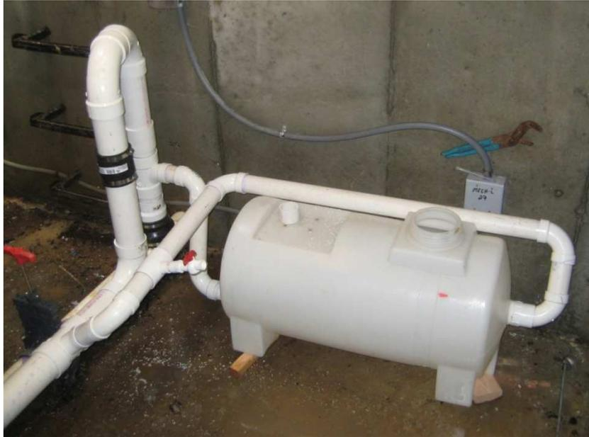
Figure 9.2: Plumbing and compositing tank
