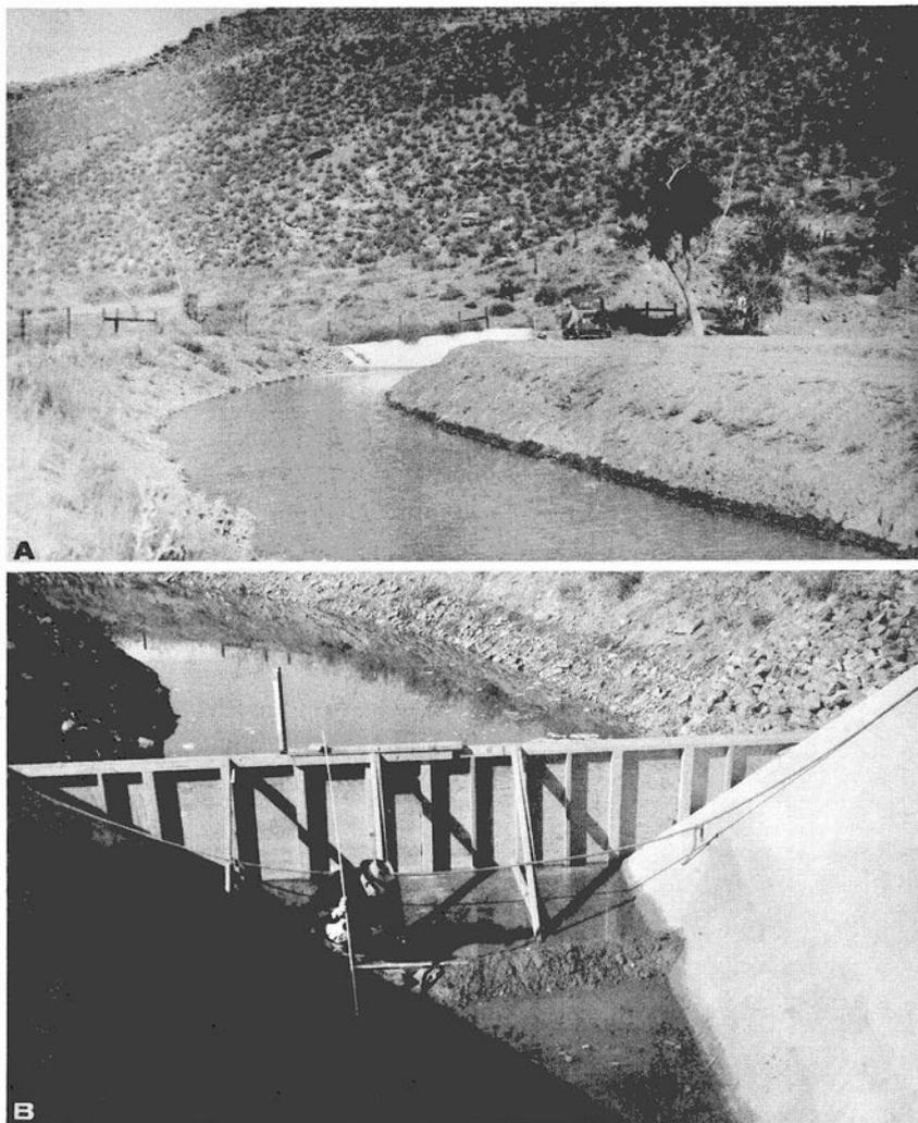
FIGURE 16.—A, Lower part of pool used for a ponding test made on the North Poudre Supply Canal in 1953 to check data from well-permeameter tests; B, bulkhead across lower end of pool.
