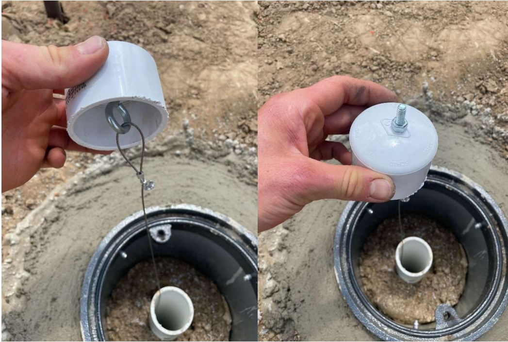
Figure A.2 Example of eyehook attachment to 2" slip cap.
