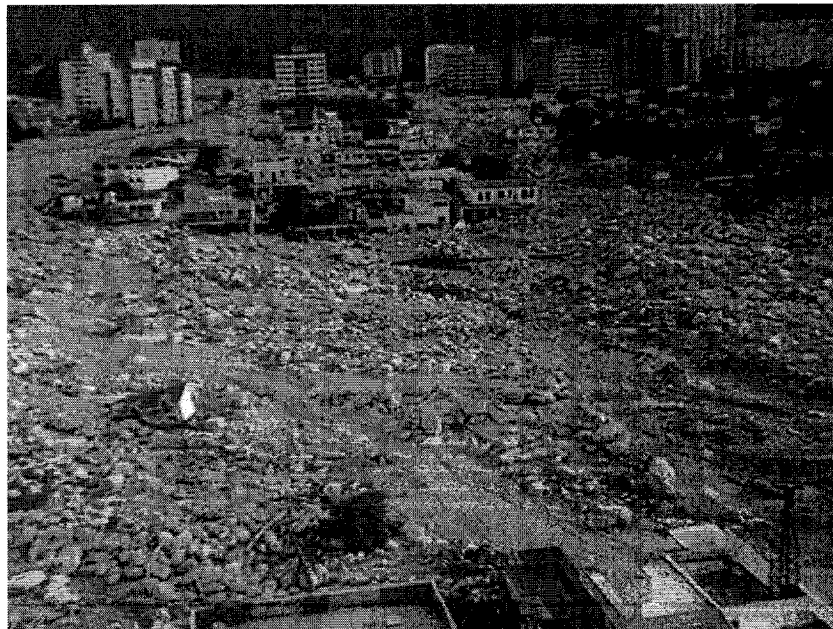
Figure 6.12: View of road damaged in Los Corales, Leon and Rojas, 2000 (personal communication)
