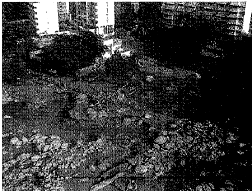
Figure 6.14: View of road damaged in Los Corales, Leon and Rojas, 2000 (personal communication)
