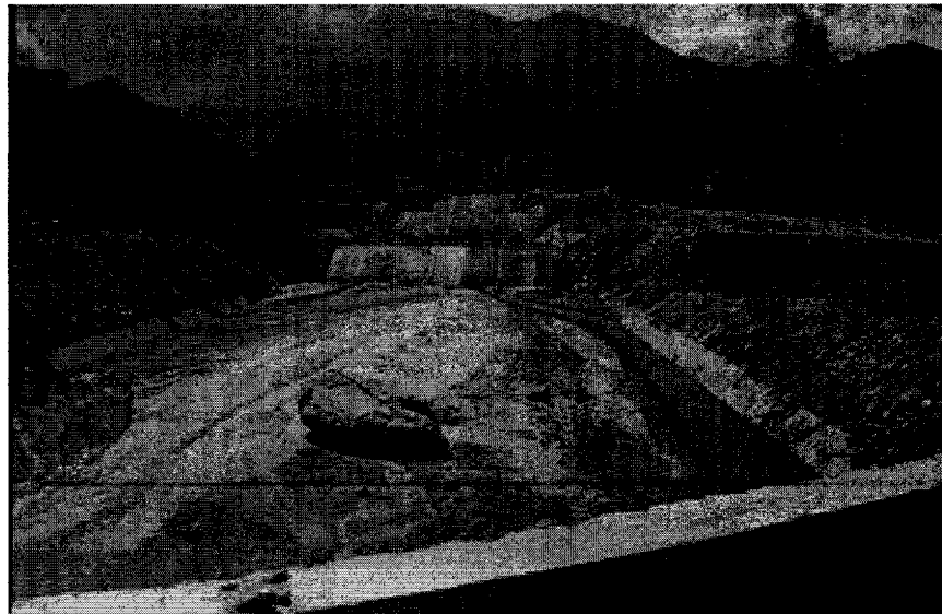
Figure 6.20: Control canal for debris flow at the Saint Julian Ravine, Leon and Rojas, 2000 (personal communication)
