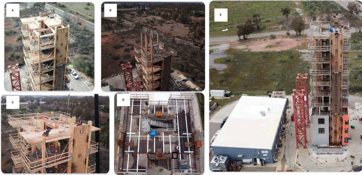
Figure 25: Final Stage of Construction of NHERI Tallwood Specimen
