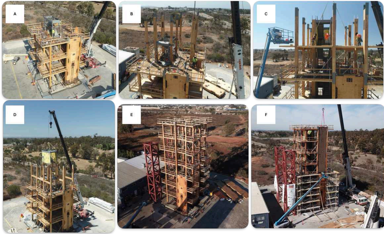
Figure 24: Construction of Floor 4 to Floor 8 of NHERI TallWood Specimen
