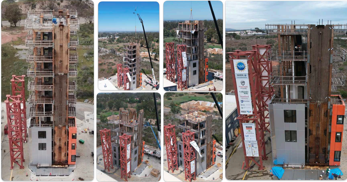
Figure 26: Overview of Deconstruction of NHERI TallWood Specimen to NHERI Converging Design Specimen.
