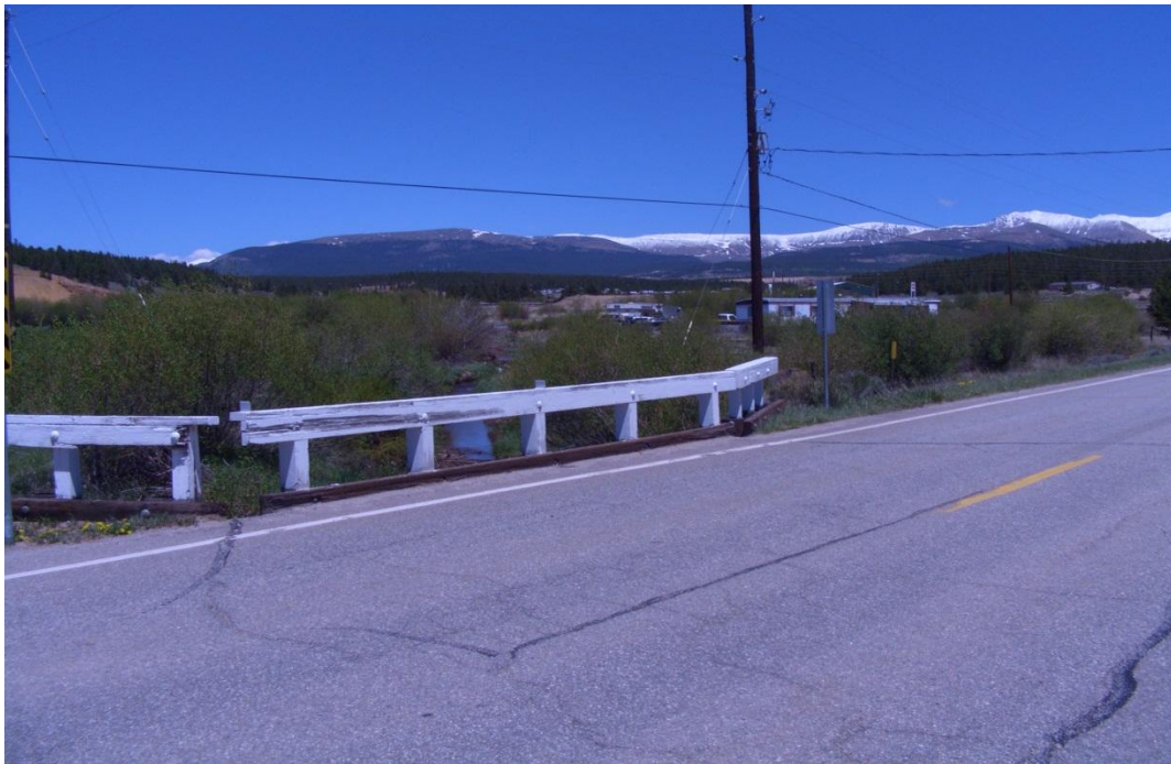
Figure C-52: County Road 5 crossing of California Gulch looking upstream (northeast).
