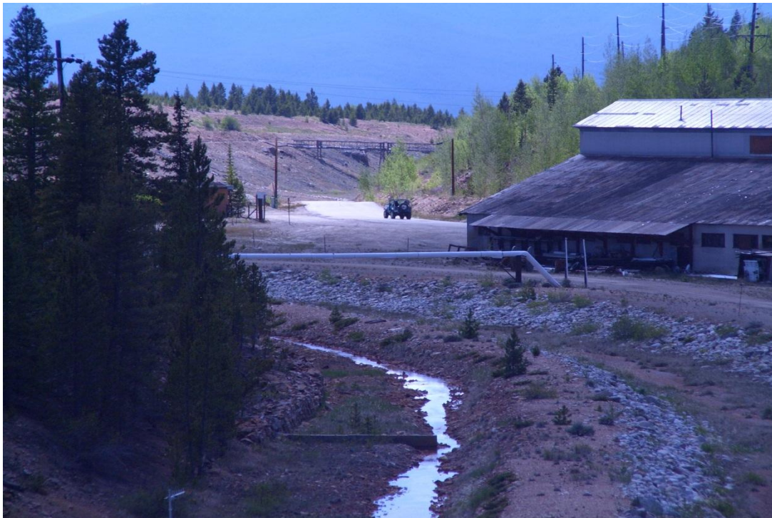
Figure C-10: View looking downstream at double channel in California Gulch near Yak Tunnel Portal below CG-1 gauge. Flow from the Yak Tunnel is collected from the left channel and delivered to the treatment plant approximately one-half mile downstream. Flow from the upper California Gulch (there is none in this photo) bypasses the treatment plant via the channel at right.
