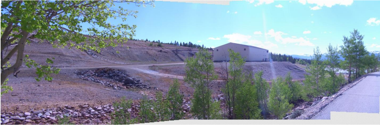
Figure C-11: Yak Tunnel Water Treatment Facility. California Gulch is in the foreground. Flow is carried from the tunnel portal via the pipeline on the far embankment.
