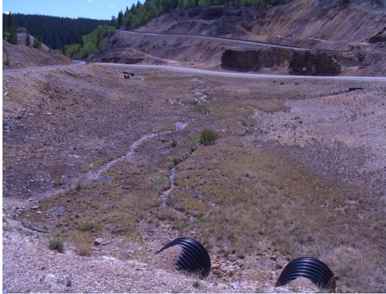
Figure C-3: Culvert outlet below Mineral Belt trail crossing over California Gulch. The series of rock weirs above the lined channel are visible downstream. No flow observed upstream of this point indicating that groundwater may be a source of flow here and downstream.
