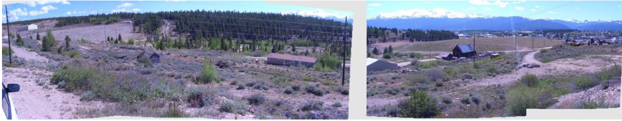
Figure C-13: Photomosaic view of Yak Tunnel Treatment Pond (left) and Apache tailings impoundment (right). Flow from California Gulch is passed in a lined channel to bypass each of these features.
