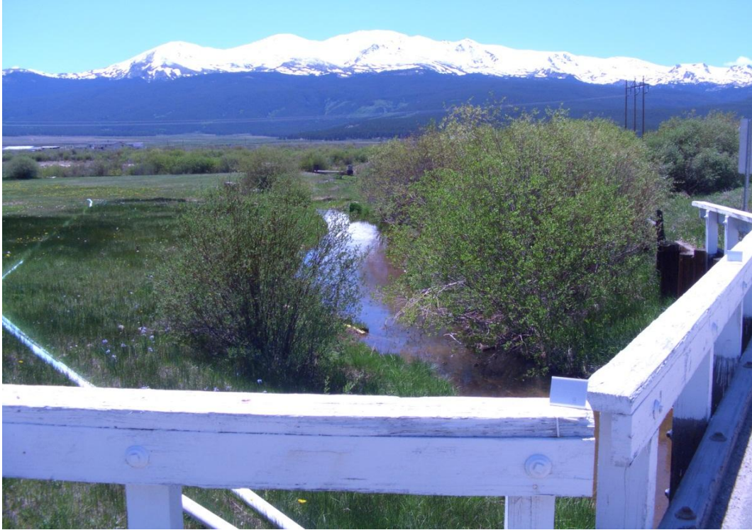
Figure C-53: County Road 5 crossing of California Gulch looking downstream (southwest).
