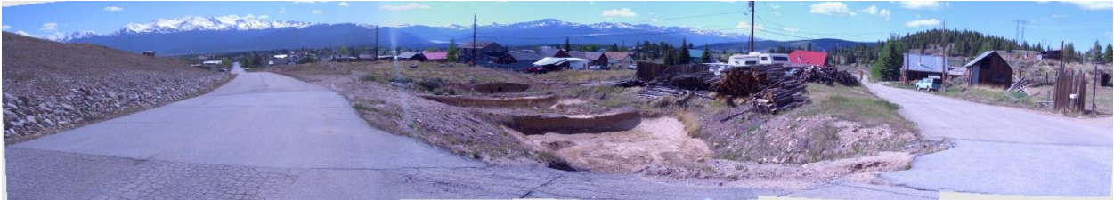
Figure C-66: Stray Horse Gulch looking downstream. Flow from Stray Horse Gulch is intercepted by the Starr Ditch and conveyed south (left) along the eastern edge of Leadville to California Gulch.
