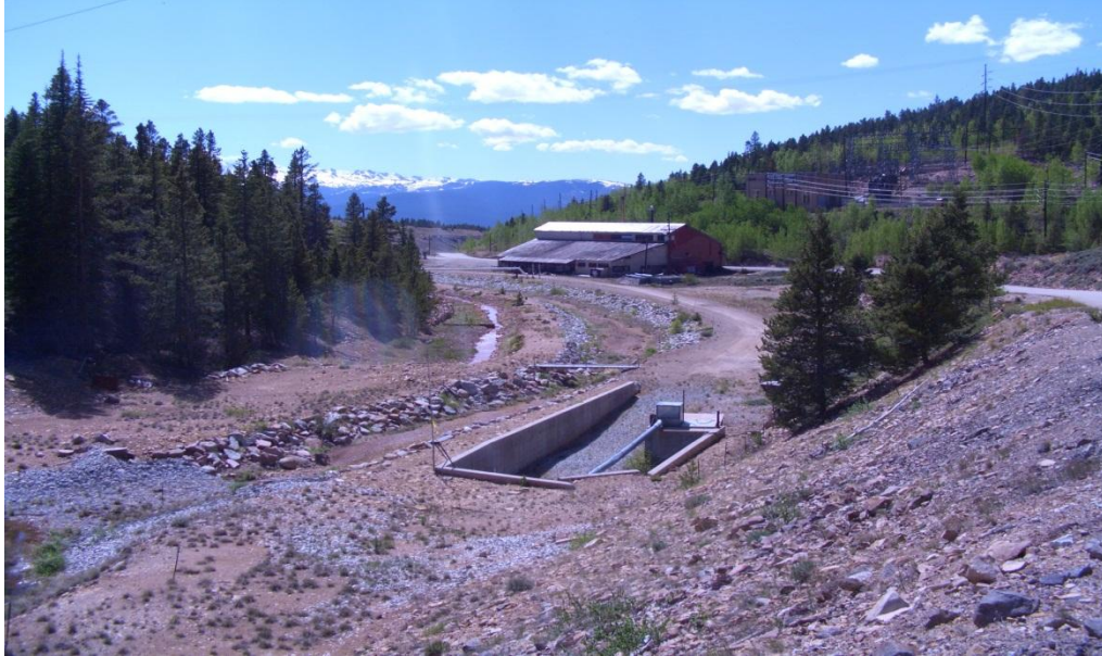
Figure C-7: View looking downstream at double channel in California Gulch near Yak Tunnel Portal below CG-1 gauge. Flow from the Yak Tunnel is collected from the left channel and delivered to the treatment plant approximately one-half mile downstream. Any flow from upper California Gulch (there is none in this photo) bypasses the treatment plant via the channel at right. Defunct flume is obscured but the foot bridge shows that its location is just upstream of the Yak ditch.
