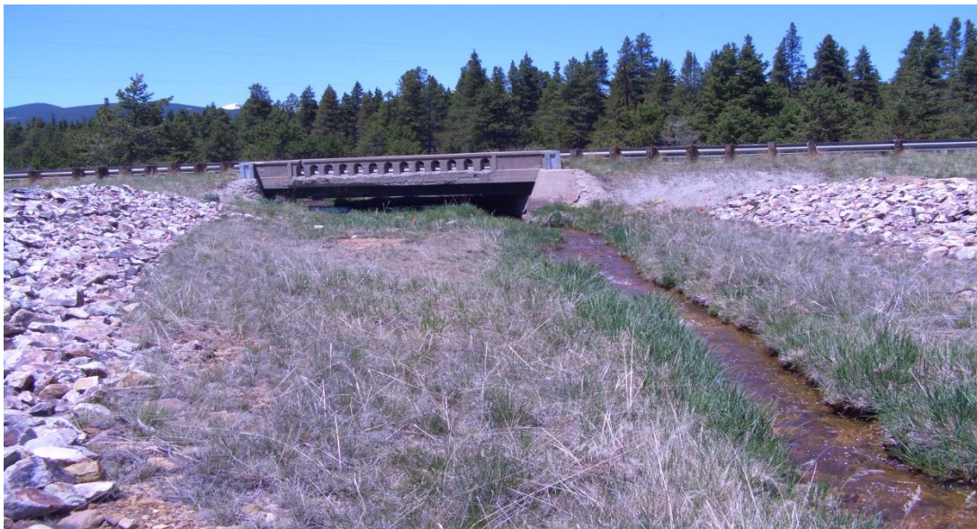
Figure C-42: US-24 bridge over California Gulch.
