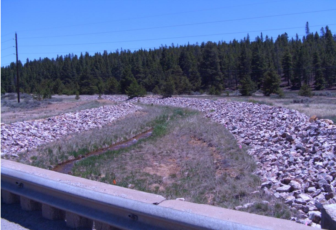
Figure C-41: Looking upstream from US-24 bridge over California Gulch below CG-5.
