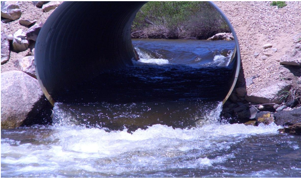
Figure C-64: Arkansas River at County Road 4. Close-up view of east culvert outlet.
