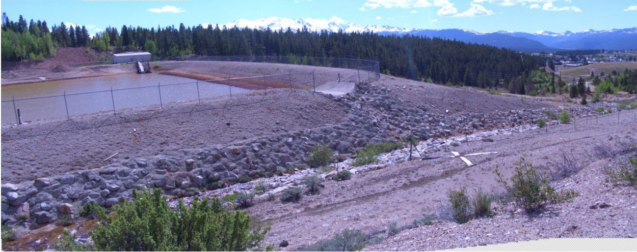
Figure C-12: Yak Tunnel Water Treatment Plant reservoir. Flow in foreground is California Gulch with Yak Tunnel Treatment Plant discharge included.
