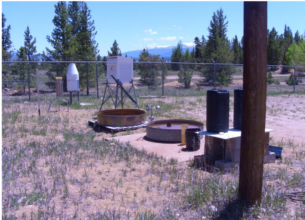
Figure C-68: Bureau of Reclamation meteorological station at Sugarloaf Dam.
