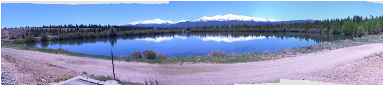
Figure C-44: Leadville WWTP final oxidation pond looking west toward Mt. Elbert (left) and Mt. Massive (right).
