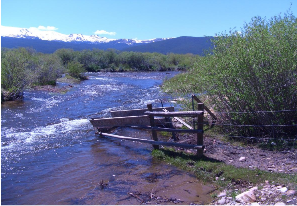
Figure C-57: AR-3A looking upstream.
