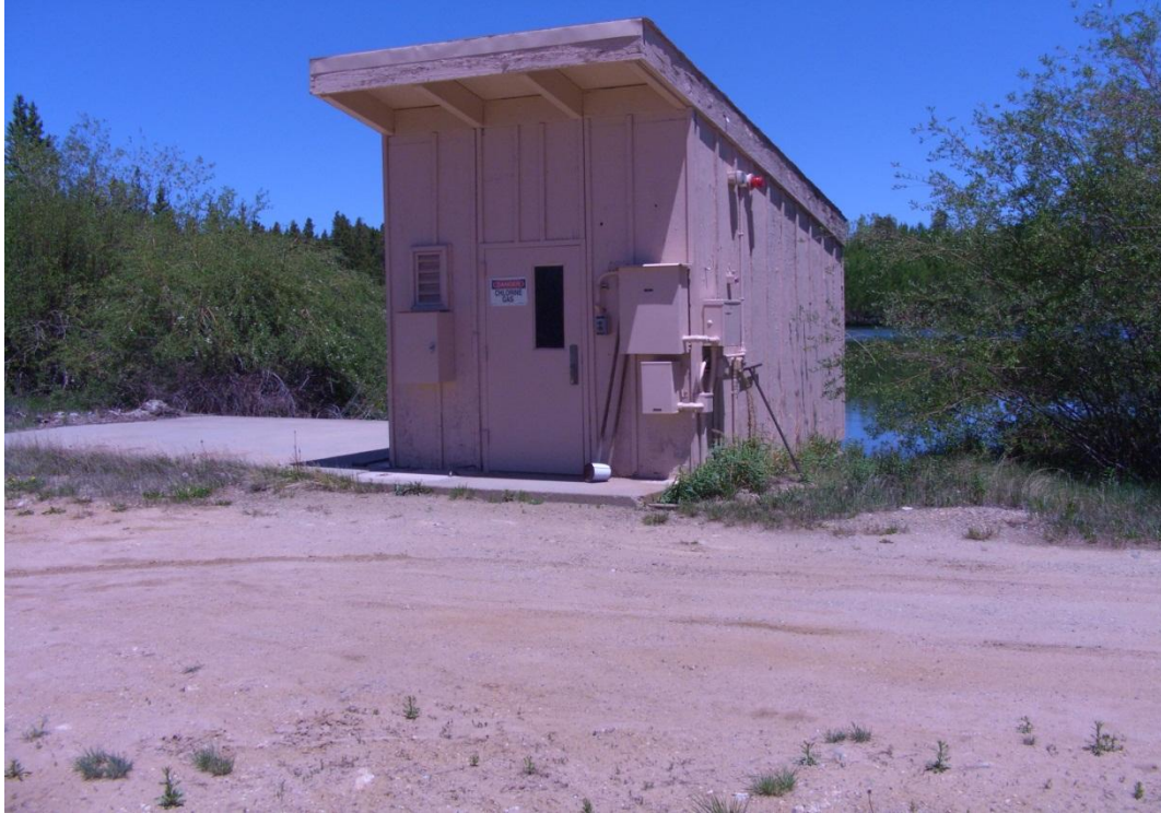
Figure C-45: Chlorination Building at outlet of oxidation pond. Chlorination is the last treatment step before water is discharged to California Gulch below CG-5.
