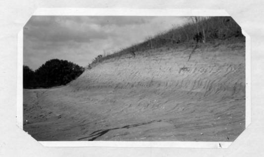
which shows material removed from borrow pit number one as applied to the project. Note the distinct difference in the shade and compact qualities of the two soils at this point.
