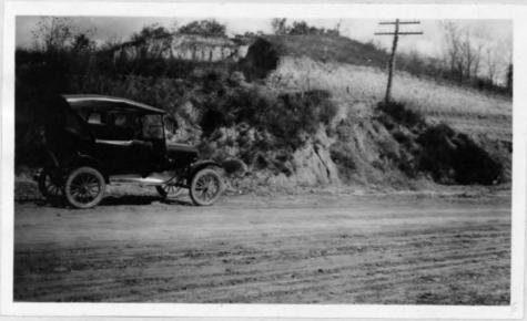
Borrow pit number one is shown by pictures number 6 and 7. The hill shown here was of a good quality of clay and the material removed was all used as surfacing material. Picture 6 will illustrate the advantageous location of the material for trapping. The depth of the surfacing material can easily be seen from picture 8,
