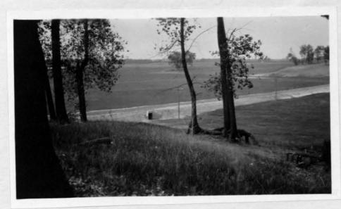
Picture number 12 shows the concrete box culvert at station 13+60-A. This illustrates very well the type of concrete work an this project. The concrete has a dense appearance, is free from board marks, and the edges are all straight, clean lines.
