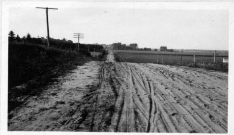
in the direction of increasing stations. This was the condition of the road before any work was done and shows the very sandy condition of the soil. The hill in the foreground was cut considerably to make the fill at the bottom.
