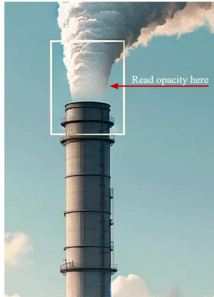
Figure 3.2: A demonstration of how to properly read opacity's from a smokestack. A common misconception is to read the opacity from the cloud, however, it's imperative that it is read at the top of the smoke stack, immediately after emission.
