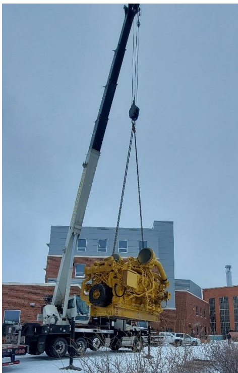
Figure 57. Crane lifting G3516J engine off a semi-trailer and placed in the back of the laboratory.
