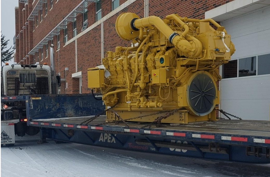
Figure 56. G3516J engine arrival at the CSU Powerhouse facility.
