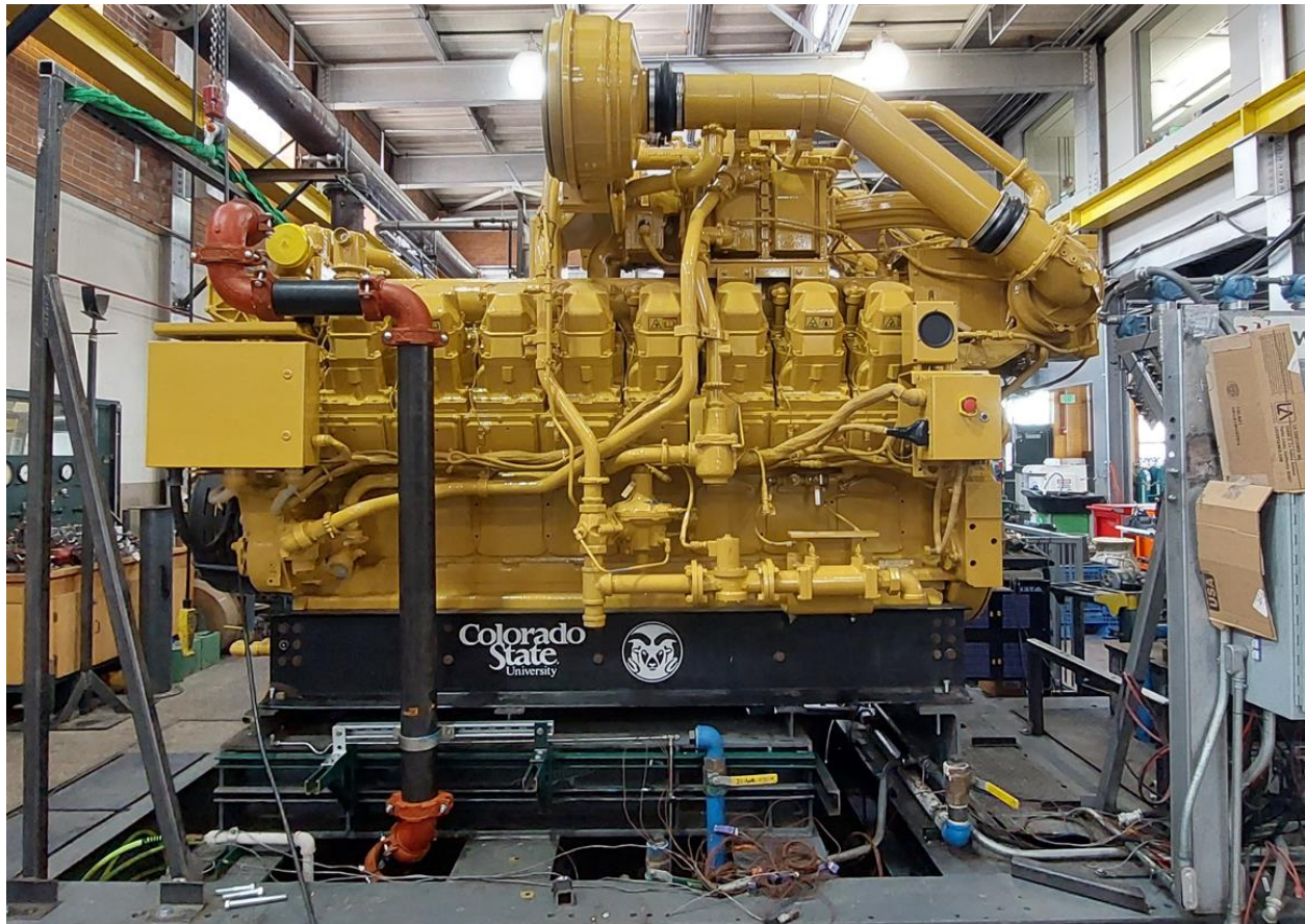
Figure 59. G3516J engine on the test bed.
