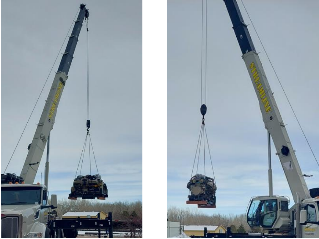
Figure 52. Crane lifting QSK50 onto a semi-trailer.
