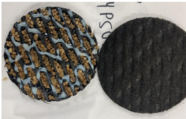
Figure Ab6. Top view of a laboratory gypsum-amended NOBB during assembly. Loctite E-120HP Hysol Epoxy Adhesive is placed on top of the geonet and the geotextile is prepared to be securely glued on top to completely reassemble to NOBB.
