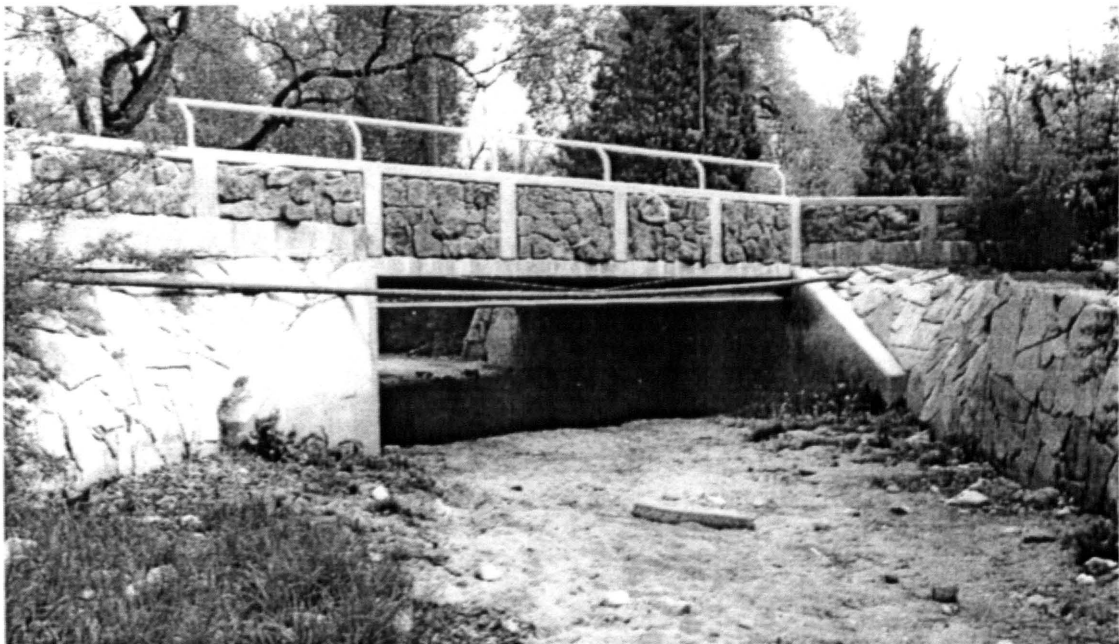
Figure 17. The New Bridge at Bryan and City Park Drive, 3 May 1986.
