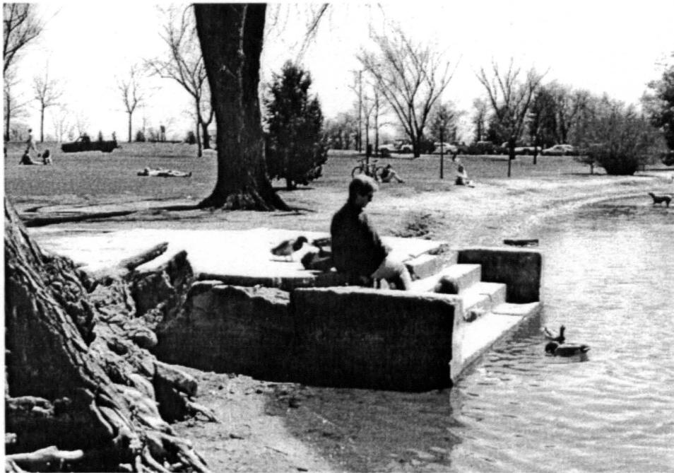
Figure 25. Concrete Steps, Remnants of the Skating House in City Park, April, 1996.
