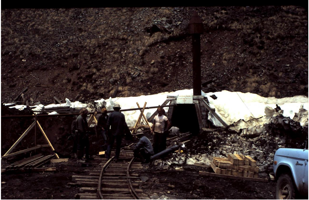
Terry Tunnel entrance. William R. Jones, June 11, 1978.
