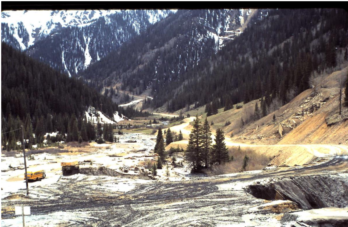
Facing downstream northwest from the entrance to the American Tunnel. William R. Jones, June 5, 1978.
