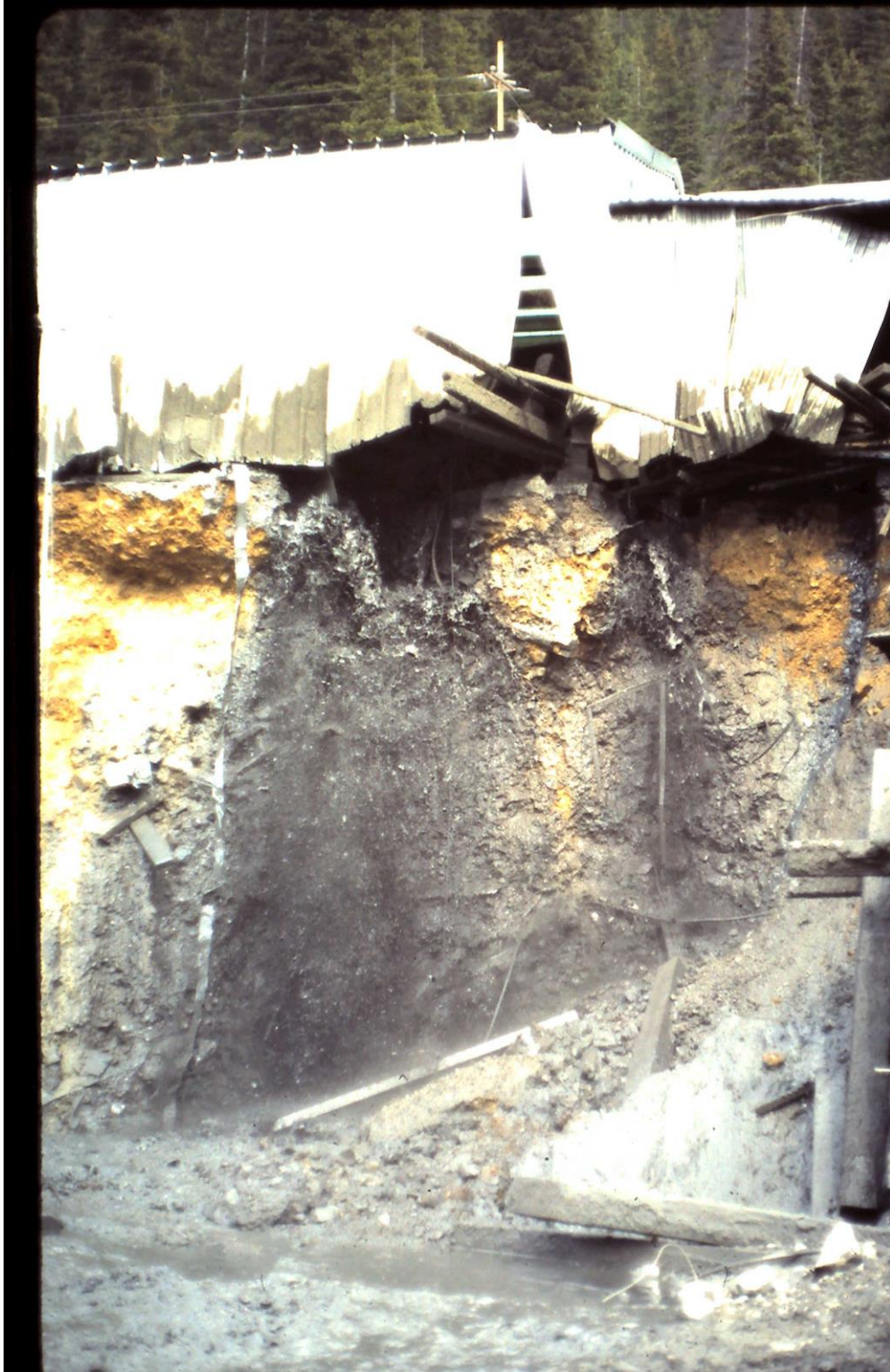
American Tunnel discharge point. William R. Jones, June 5, 1978.
