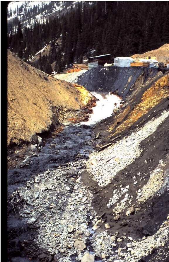
Figure 4: Photos taken at Gladstone and the American Tunnel the day after the flood. A) mine structures were damaged and a large amount of black mud was deposited. Photo is taken from immediately west of the American Tunnel entrance facing upstream. B) Gravel and black mud were deposited and a channel was sharply incised just downstream of the mine. Photo is taken looking downstream toward the entrance of the American Tunnel. Photographs courtesy of Bill Jones.
