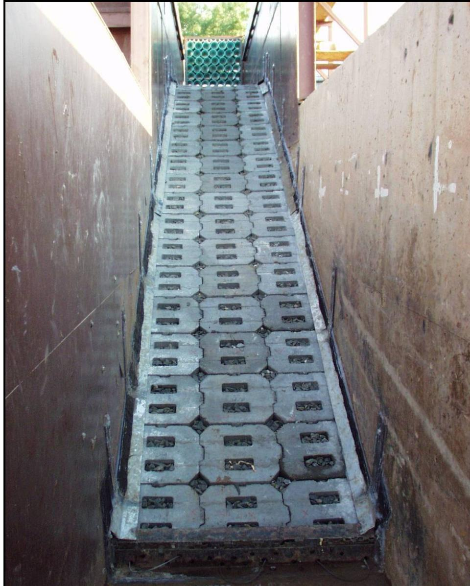
**Figure 4.2: Photograph of Installed Petraflex Blocks**
