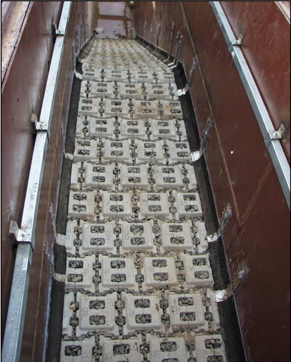
**Figure 4.1: Photograph of Installed 30S Blocks**
