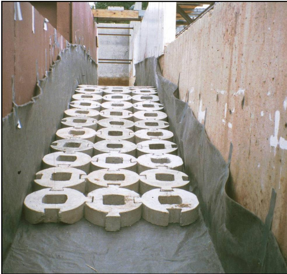
**Figure 4.3: Photograph of Corps Blocks Installation**
