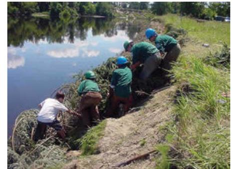
*Workers along the Connecticut River as it passes through Fairlee, Vermont, United States. During the summer of 2002 a restoration project aimed at restoring a severely eroded riverbank utilized overgrown Christmas trees to create a revetment at the work site. The trees were eventually planted with various aquatic plant life to help further trap sediment and prevent erosion. Courtesy of US Environmental Protection Agency*
