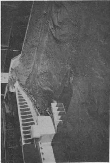
A Scour Downstream from North Abutment
