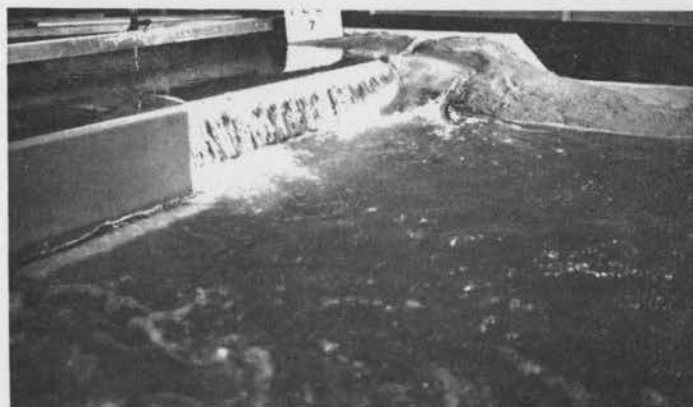
B Flow Conditions at North End of Abutment Section
