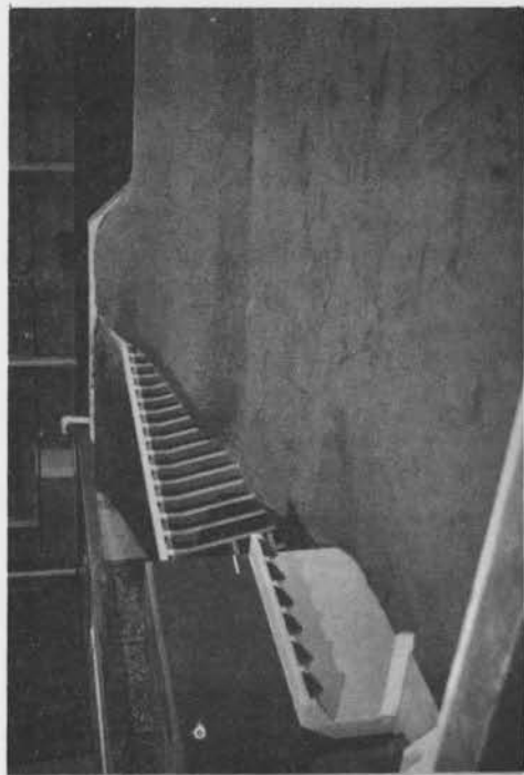
B North Bank before test
