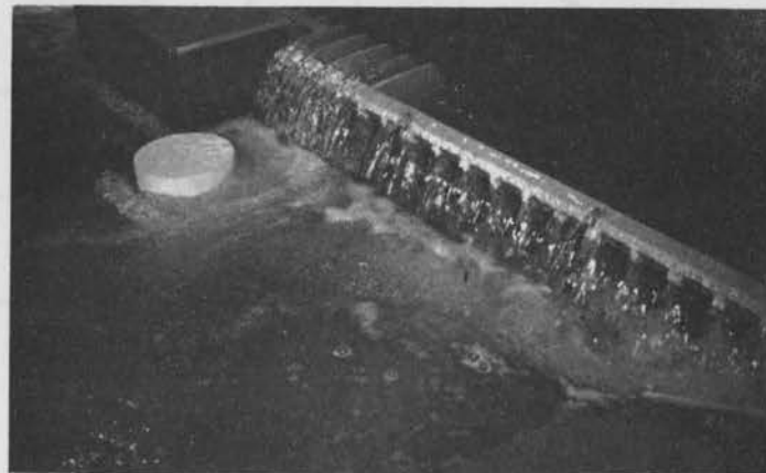
C Flow Conditions at Base of North Abutment
