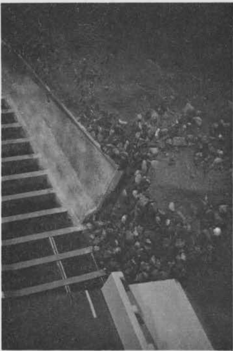
B Scour at South End of Trough
