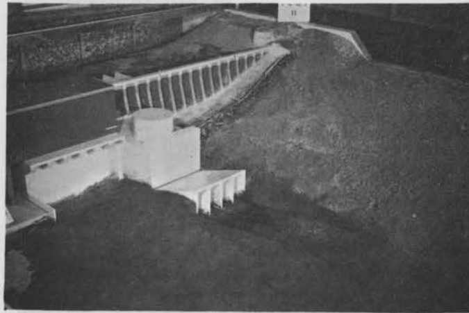
B Powerhouses and North Abutment
