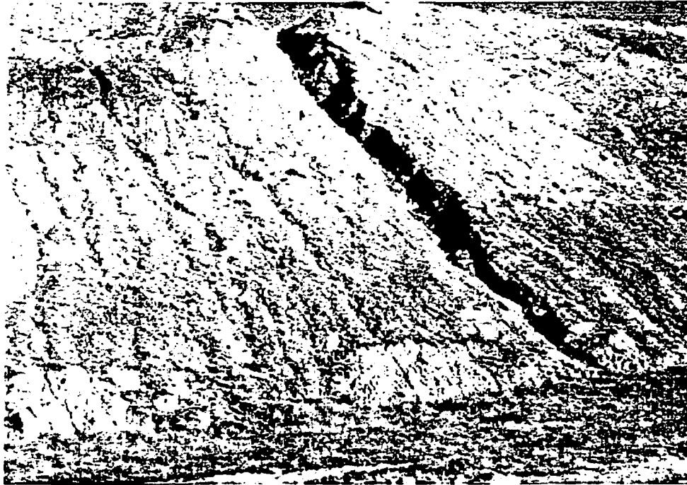
Figure 1.1 Typical Gully on Waste Impoundment
