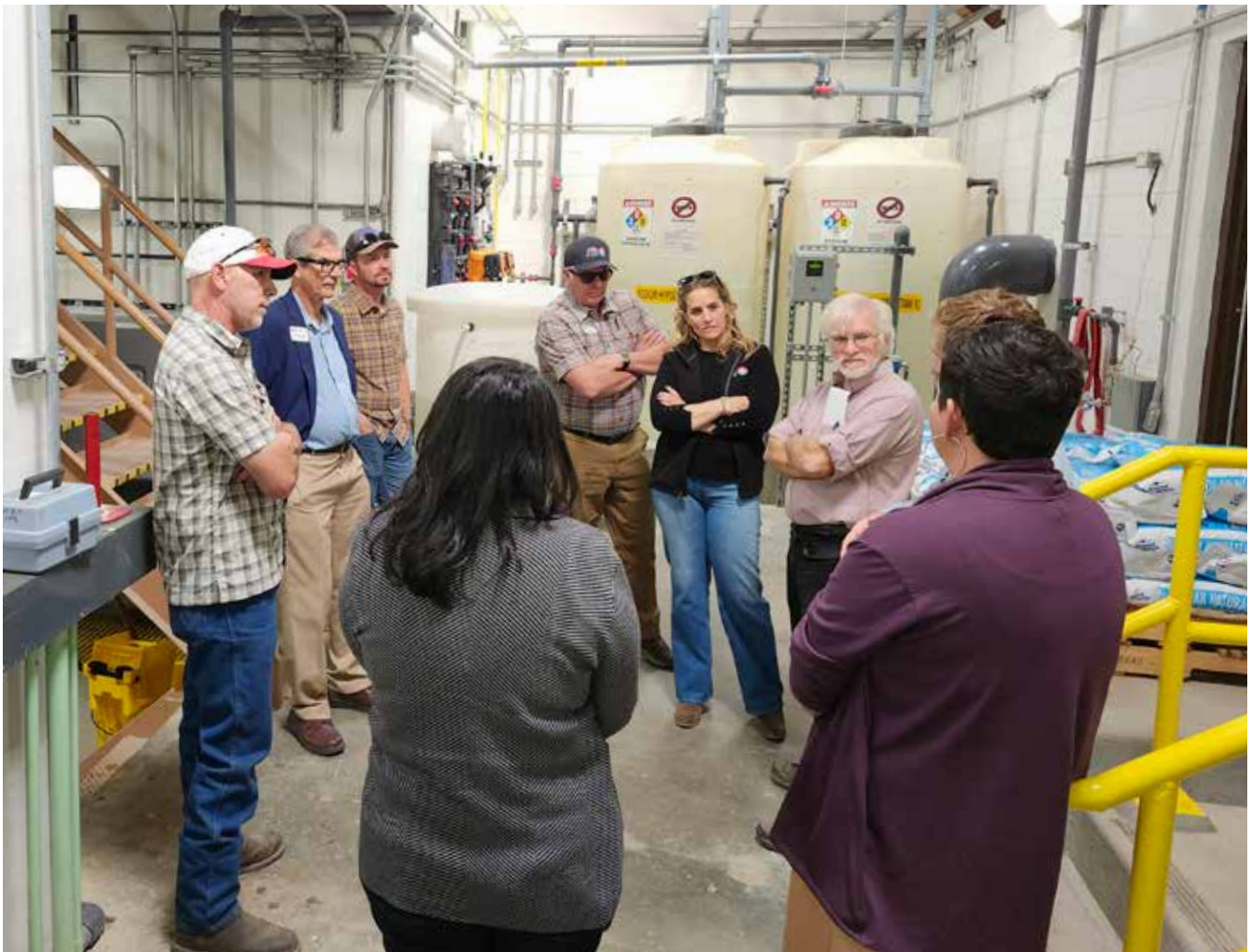
Buena Vista used EIAF grant funding for a water treatment plant expansion to secure reliable water sources to meet current and future demands. Photo courtesy of DOLA.
