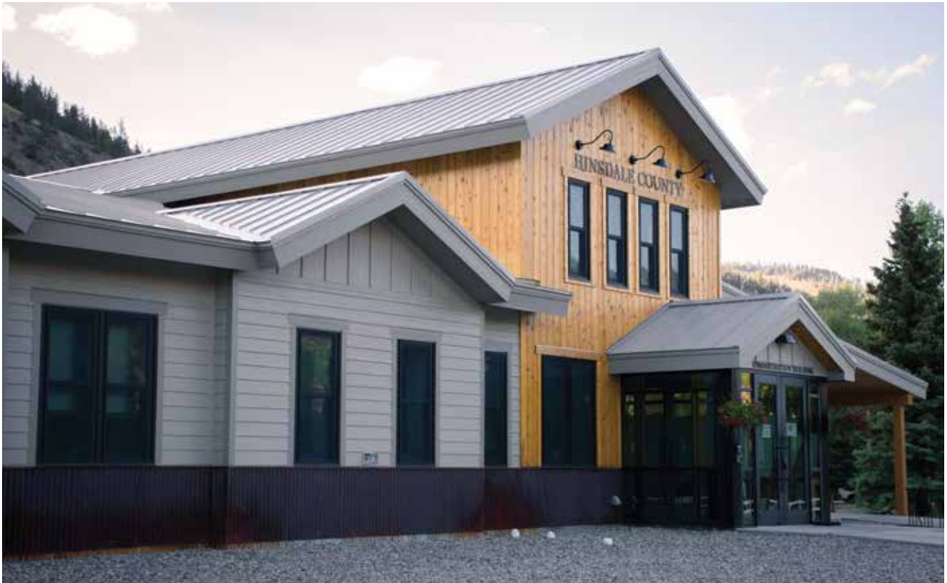
Hinsdale County received over $1 million from an EIAF grant for the new operations building. Photo courtesy of DOLA.
