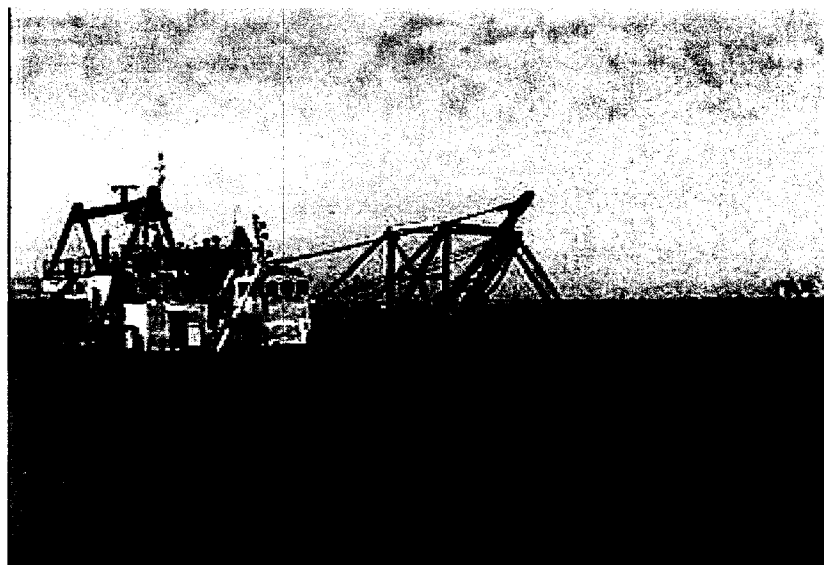
Figure 3-17. Sediment dredging on the Lower Nakdong River
