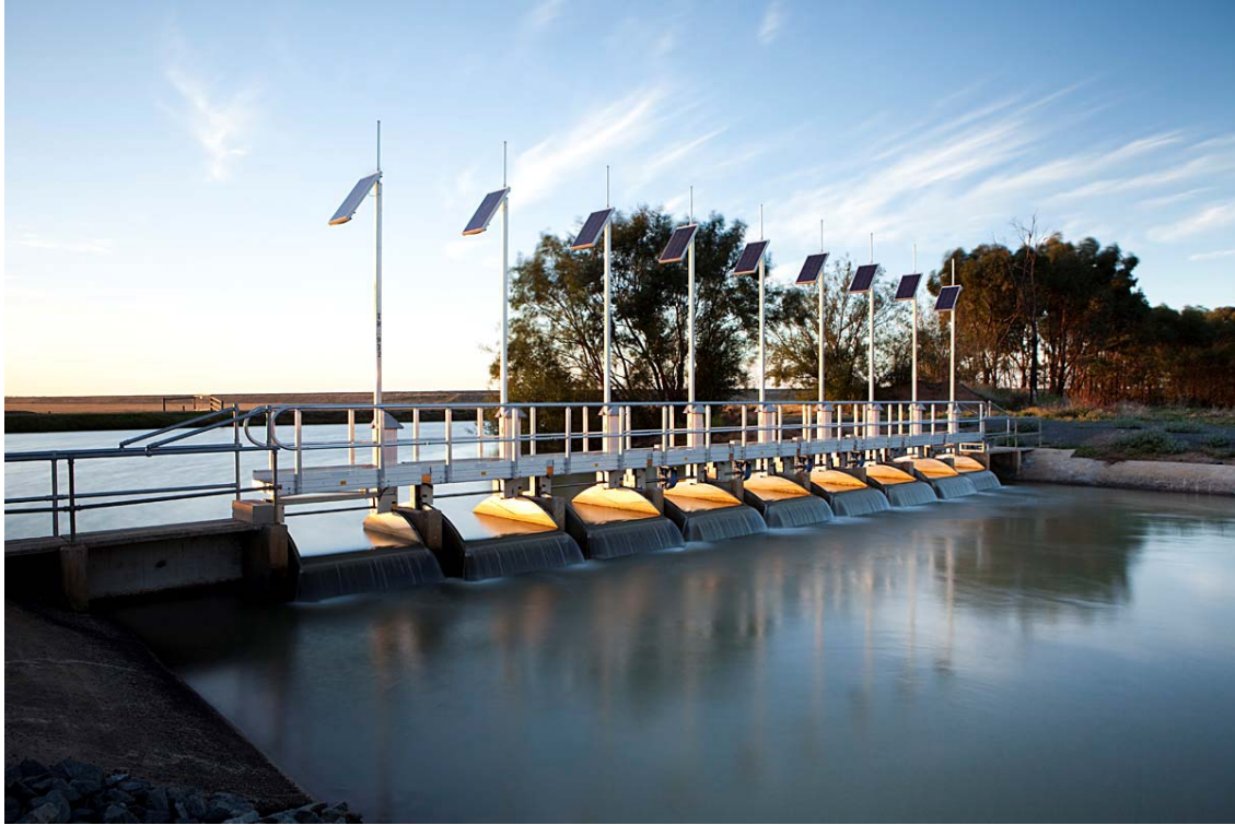
Figure 4. 9 FlumeGate™s at the CG No 8 Channel Offtake, Tatura, Australia
