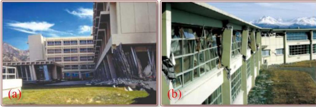
Figure 1-1: (a) Olive View Hospital damaged during the 1971 Sylmar earthquake (Çelebi et al., 2003) and (b) West Anchorage High School damage during the 1964 Alaska earthquake (Federal Emergency Management Agency, 2010).
