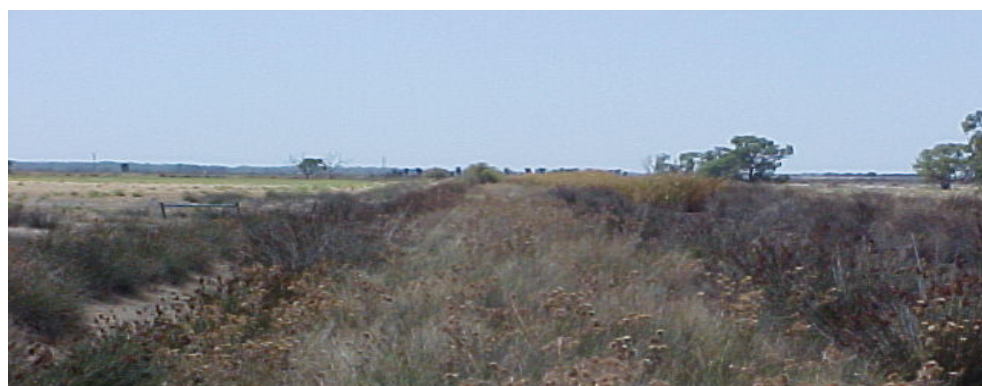
Photo 3. Low use supply channel infested with weeds
