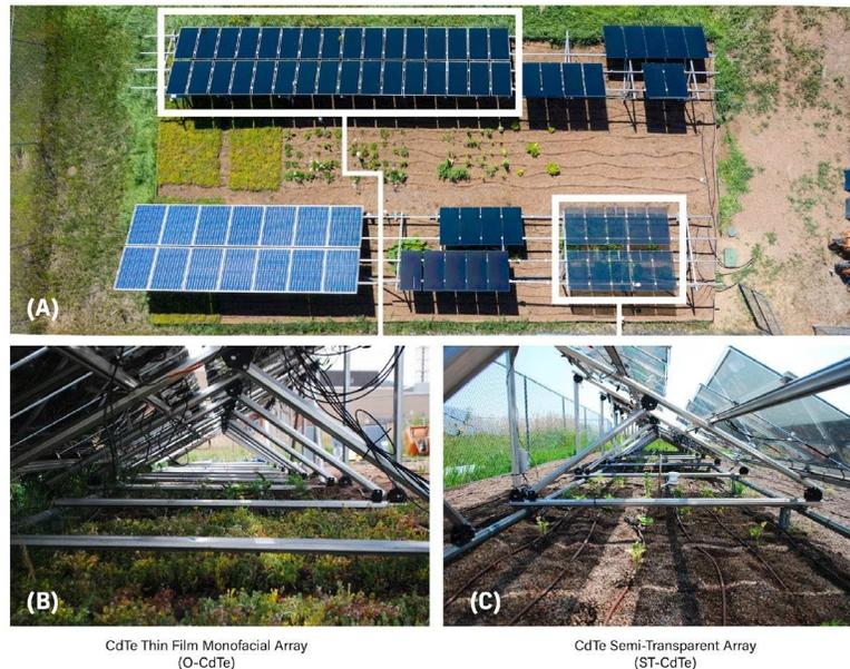
**Figure 13.** Foothills Campus site overview. **(A)** Construction emulates a RAPV installation. **(B)** Growing environment under the O-CdTe panels at Foothills. **(C)** Growing environment under the 40% ST-CdTe solar panels at Foothills.
