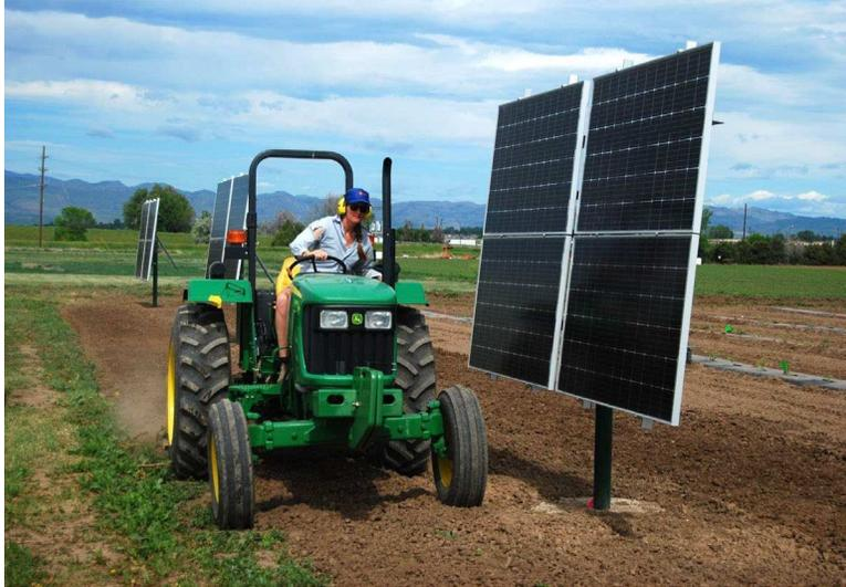
Figure 25: Array adjustability for field preparation.
