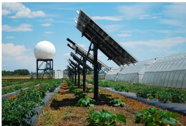
Figure 26: ARDEC South agrivoltaic research site planted with open bed in the middle row, and plastic mulch in the north and south rows.
