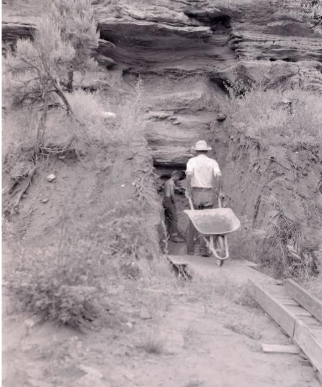
Figure 13 – Taken at the beginning of the 1949 season, this photo gives a sense of scale for the completed 1948 trench. Here 1949 crew members (David Curtis, back, and Charles Best) clean up wall-fall which occurred between these seasons. (ARC.DNM04_001_1916).
