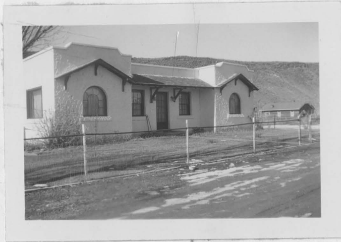
Figure 15.--SOME NEW HOMES ARE WELL CONSTRUCTED AND MODERN.
