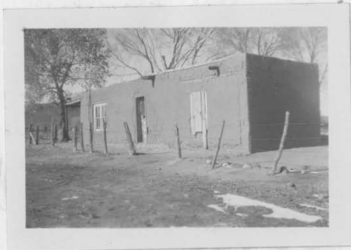
Figure 13.--MUD-PLASTERING IS COMMON AMONG THE HOMES OF PEOPLE IN LOWER-INCOME BRACKETS.
