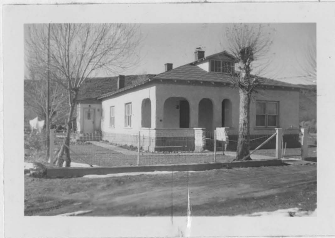
Figure 16.--GABLED ROOFS AND STUC- COED WALLS ARE TO BE FOUND IN SEVERAL NEW HOMES.
