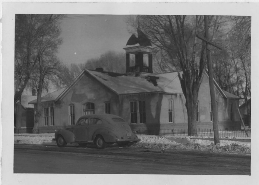
Figure 11.--COSTILLA COUNTY COURT HOUSE, BUILT IN 1883.
