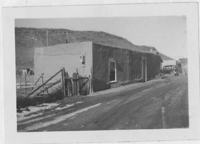
Figure 14.--ELECTRICITY HAS FOUND ITS WAY INTO OLD ADOBE HOMES.
