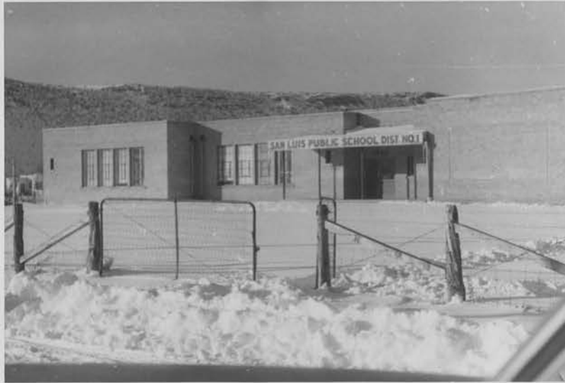
Figure 7.--ELEMENTARY PUBLIC SCHOOL BUILDING-- NEWER ADDITION.
