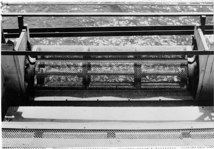
Figure 9. Rotary screen for debris removal (courtesy of W. R. Humphreys)
