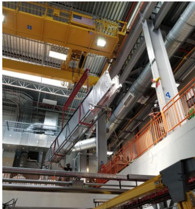
Figure 2.42: Multiple MINOS modules being transferred from the loading dock to the top of the detector via the building crane.
