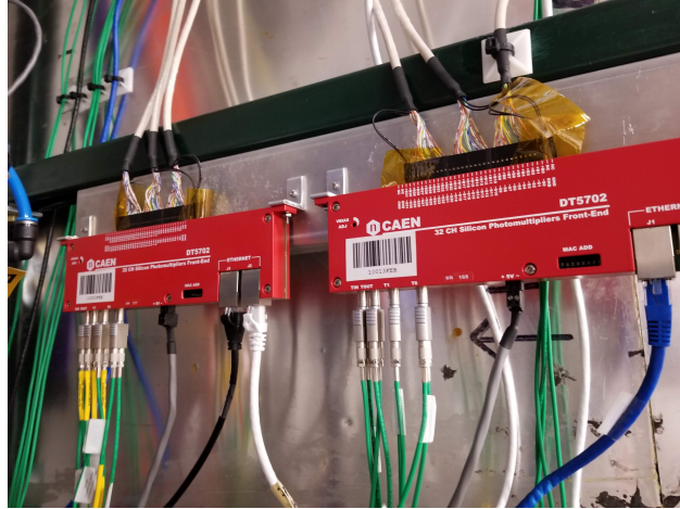
Figure 2.45: Example of FEBs once all cables were installed.
