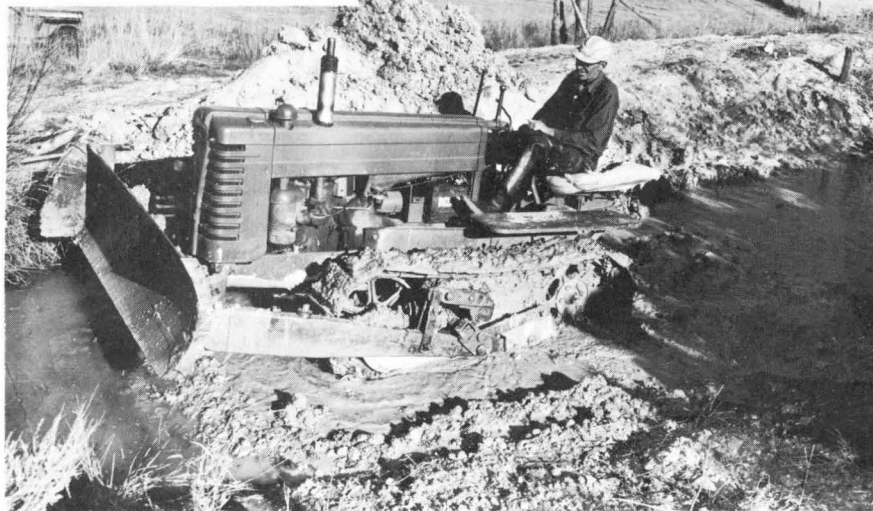
Photo 4--The bentonite can be shovelled into the water as the dam is washed out, but in some cases, as above, a small bulldozer has been used.
