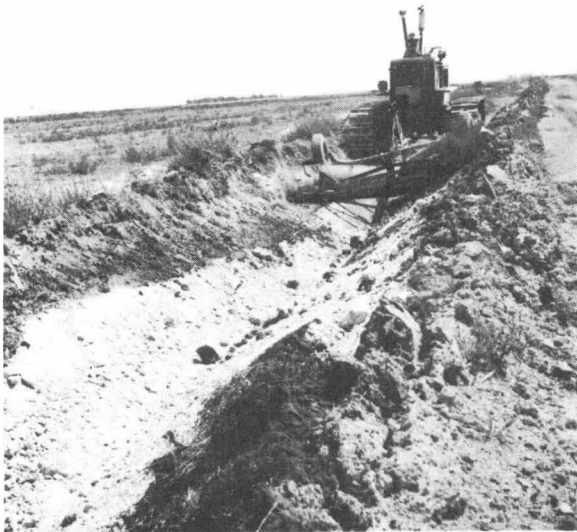
Photo 6--In several instances, the dams of bentonite have been spaced along a canal and then spread with a V-ditcher rather than with water.
