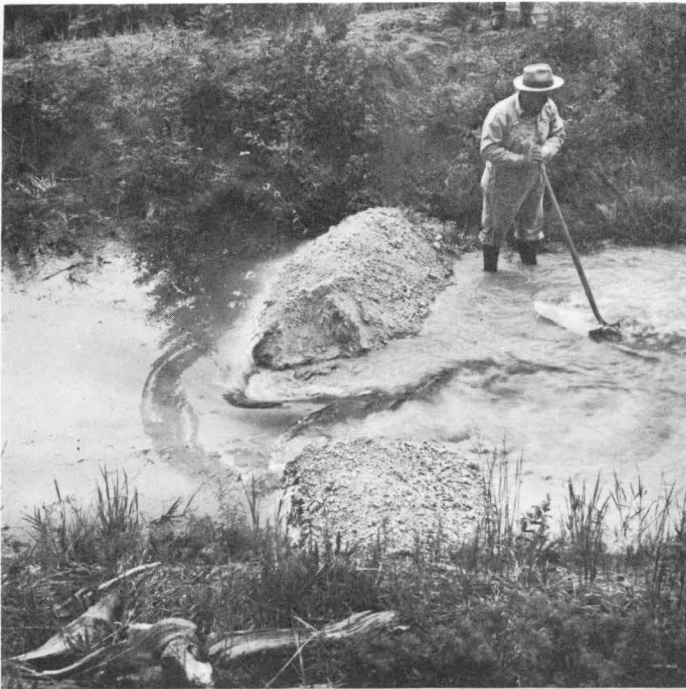
Photo 3--Most common method of application consists of placing dams of bentonite in dry canal, then running in small head of water and washing bentonite down canal.
