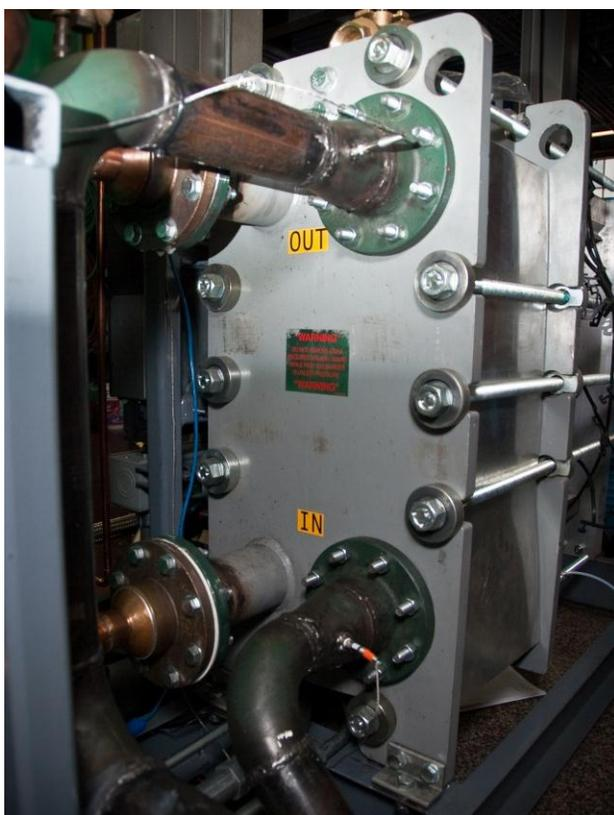
**Figure 5-2: Vaporizer as installed with piping.**
