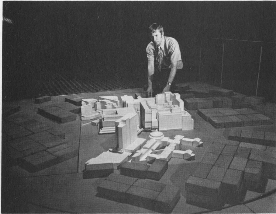
Figure 3. Model Installed in Wind Tunnel.
