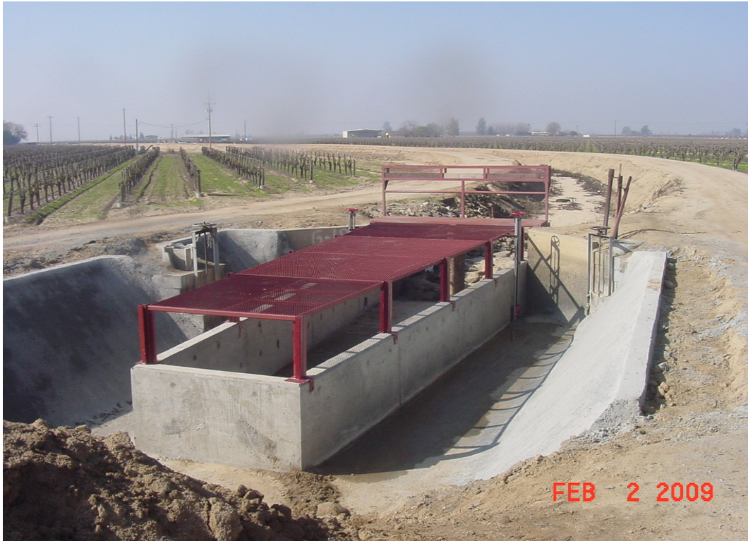
Figure 4. Weir Retrofitted with LCW
