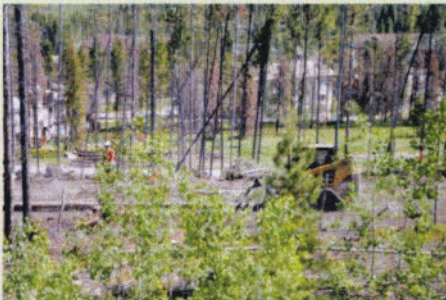
Removing trees in the railroad easement - Winter Park
