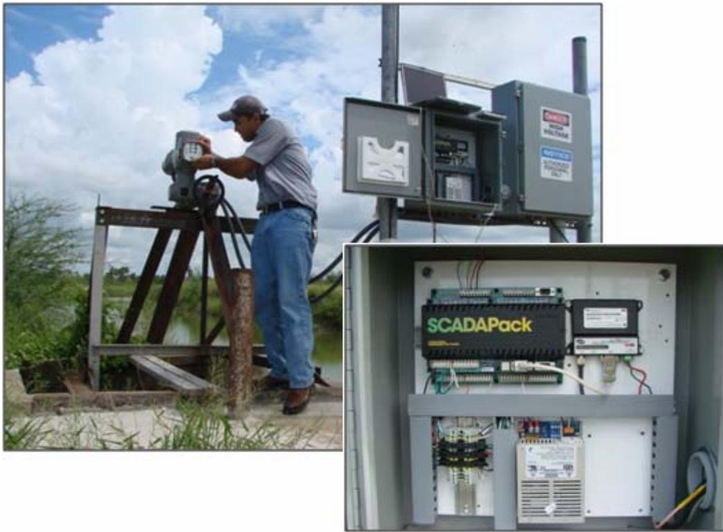
Figure 3. The Remote Terminal Unit (RTU), which consists of PLC, radio, power converter, fuses and terminals and actuator at the Emergency Gate site.
