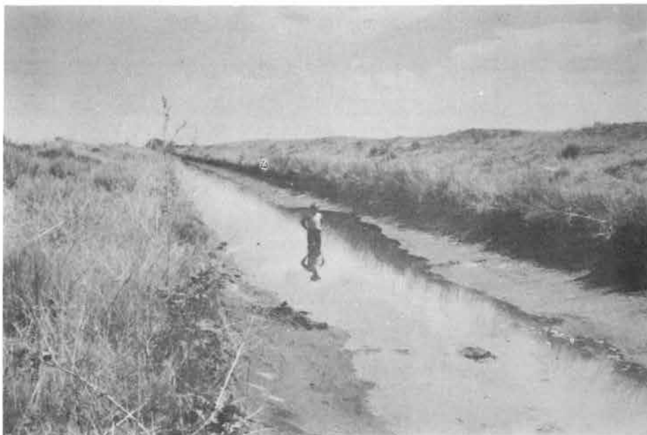
Fig. 23 Erosion of the Bed of Canal No. 1 Caused by Wave Action
