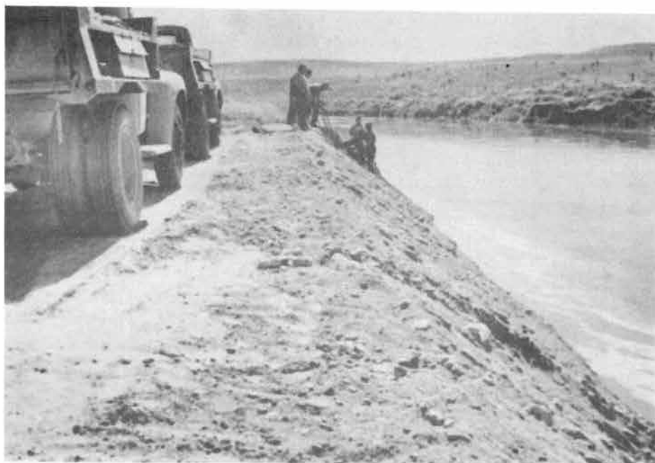
Fig. 16 Placing of Protective Material on the Banks of the Interstate Canal in Wyoming
