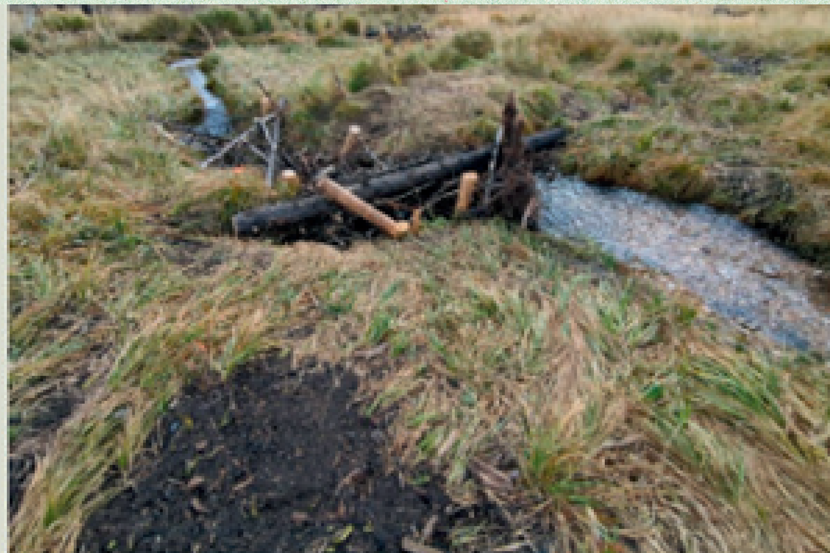
PALS installed in the Cameron Peak Burn area in the Elkhorn Creek watershed. (Photo credit: Ayers Associates)
