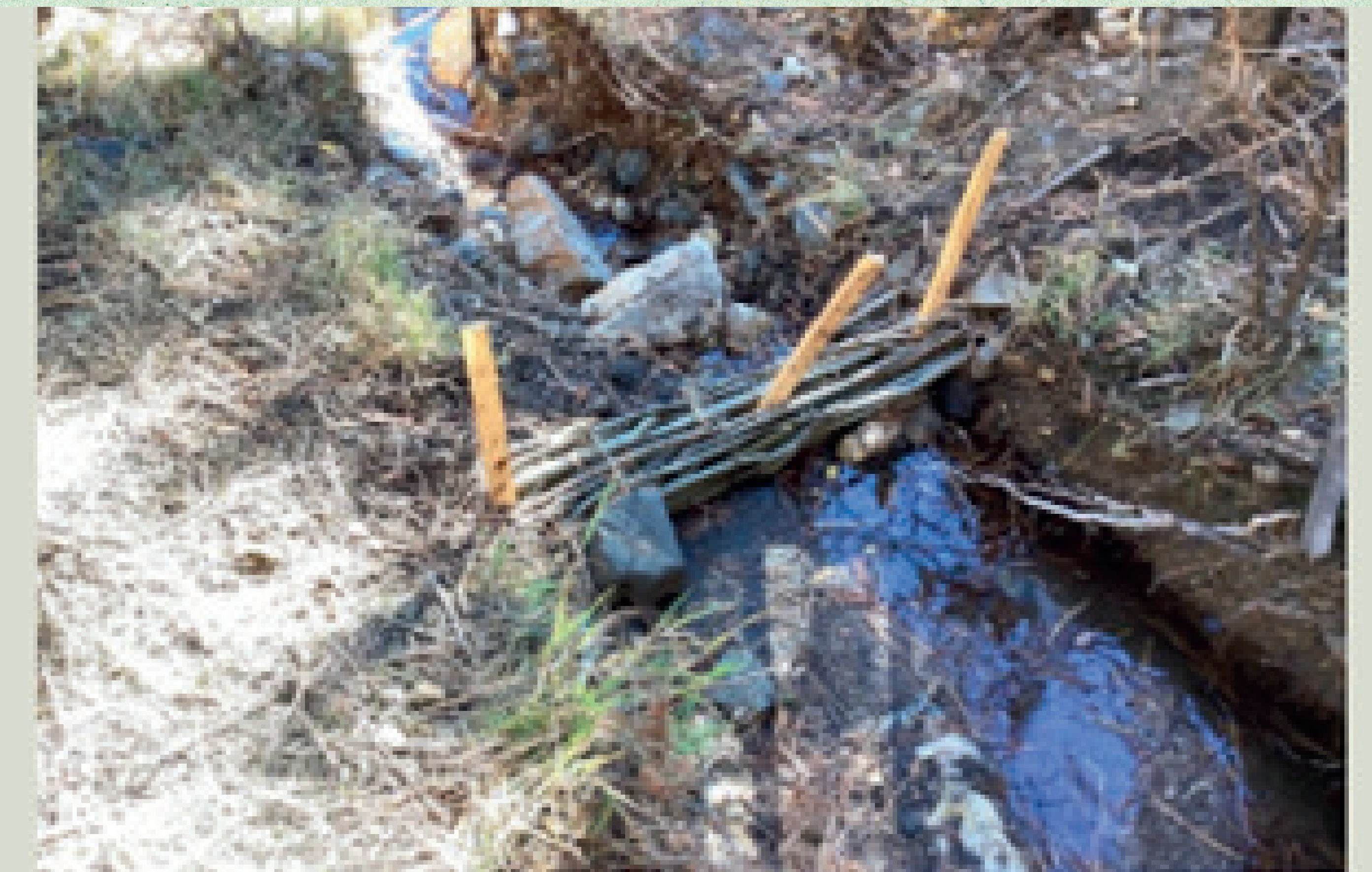
Willow wattles help to establish woody riparian vegetation. (Photo credit: Ayers Associates)
