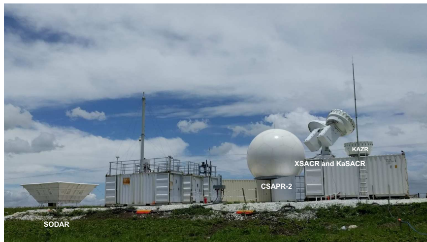
Figure 4.2: ARM mobile facility deployed during CACTI-RELAMPAGO. Sensors left to right: Sonic Detection and Ranging wind profiler (SODAR), C-band Scan Precipitation Radar 2 (CSAPR-2), X and Ka band Scan ARM Cloud Radars (XSACR and KaSACR), and Ka-band Zenith Radar (KAZR).
