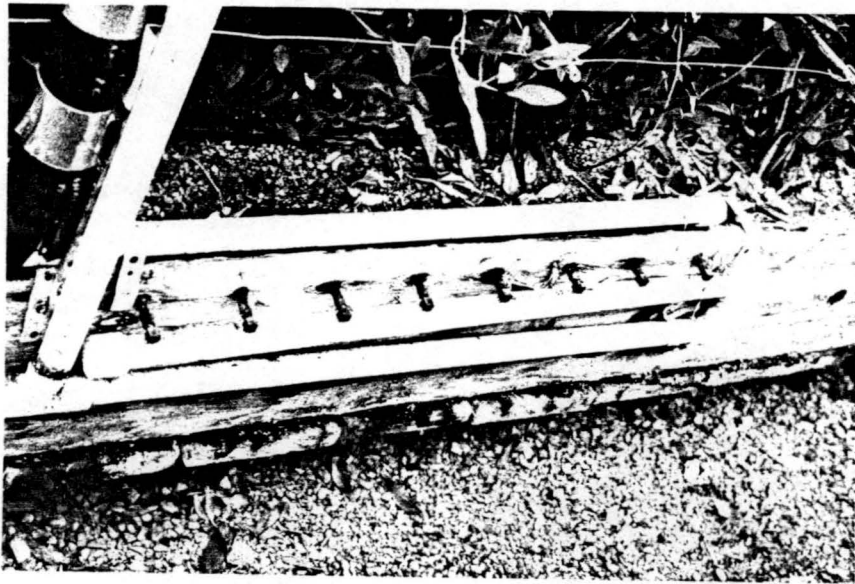
Fig. 2.3. PVC supply and return lines attached to a bench.
