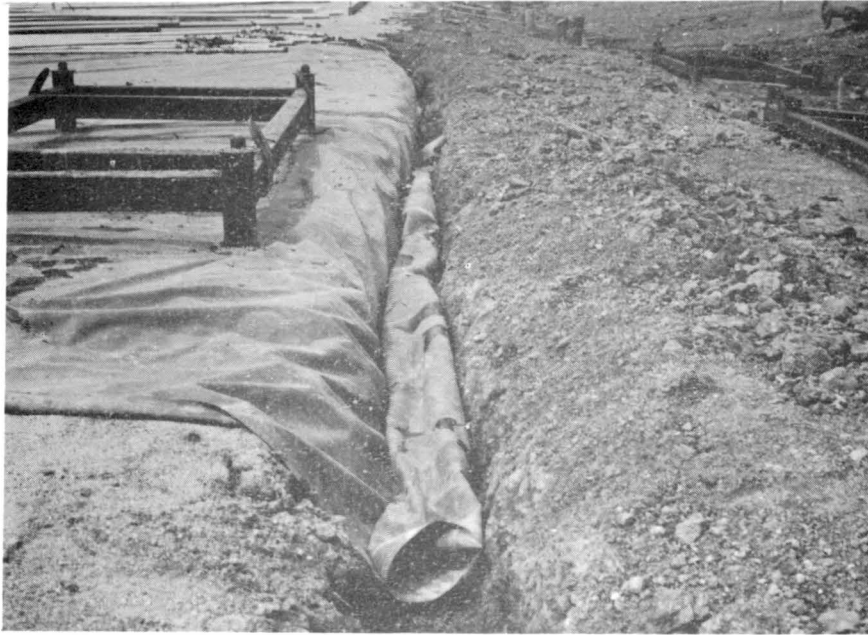
Fig. 11 - The outside of the rubber surface was buried in a small trench.
