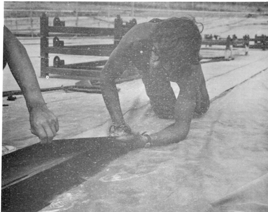
Fig. 10 - The two prepared surfaces were joined and the joint was rolled with a hand roller.
